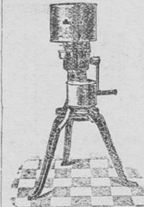
chine with self-balancing bowl. Freer action and few ball-bearings than any other machine on the market. Melotte bowl is shallow and wide and opens in the
