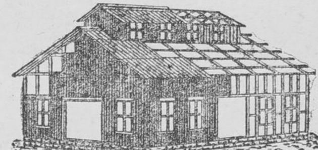
PEDLAR'S CORRUGATED IRON is made on a 36,000 m. press (the only one in Canada) one corrugation at a time, and is guaranteed true and straight to size.
