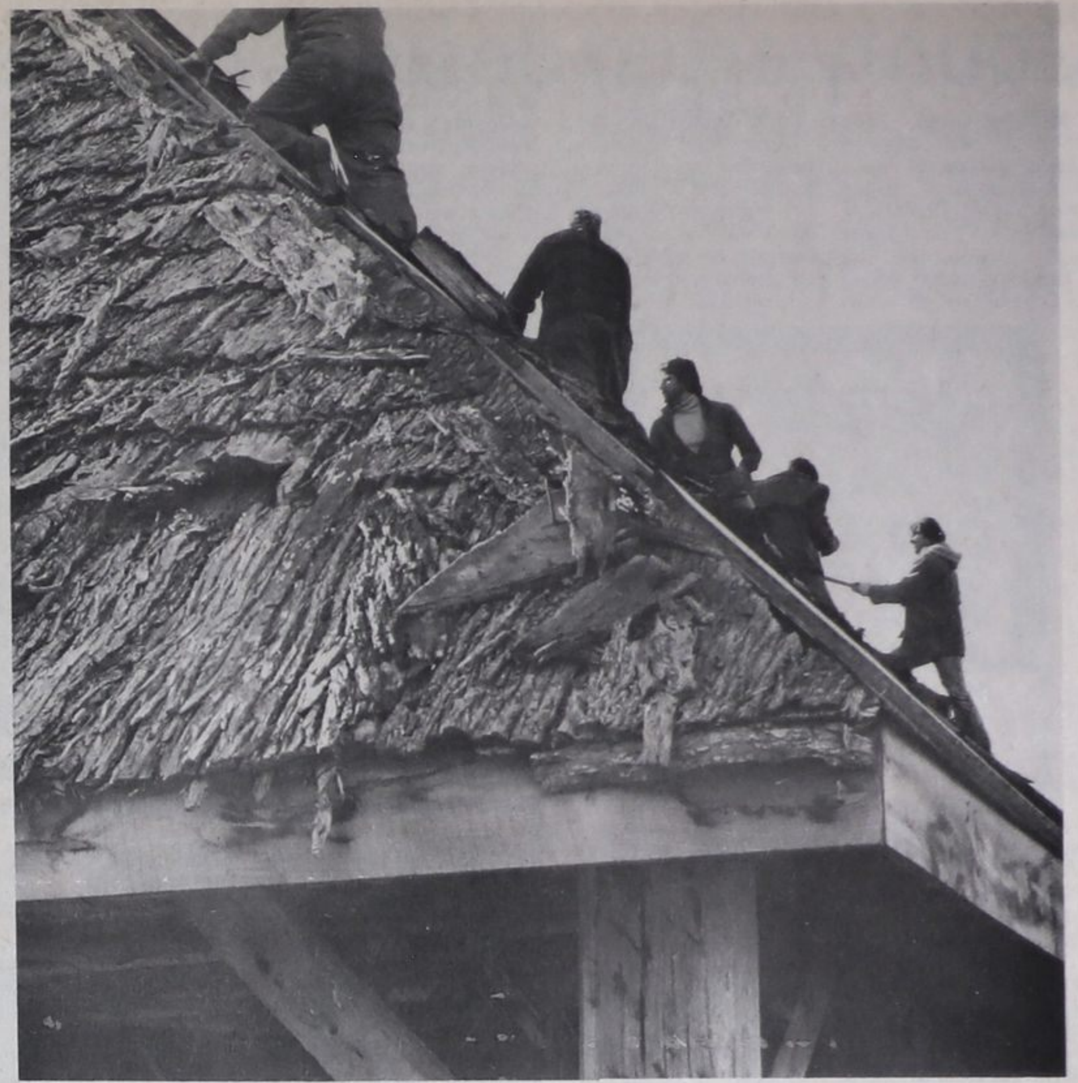
Scaling the roof
