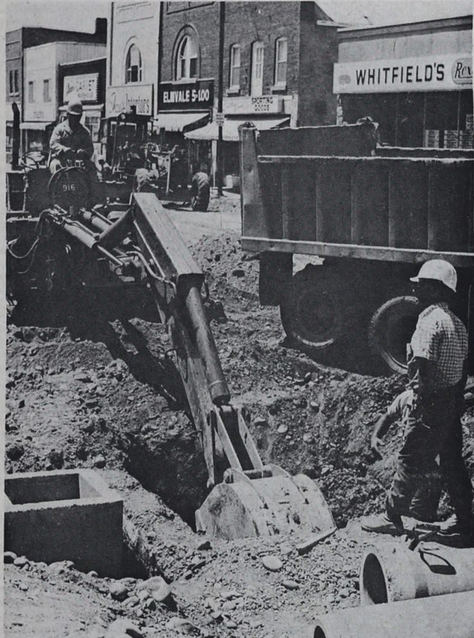
Queen St. torn up
