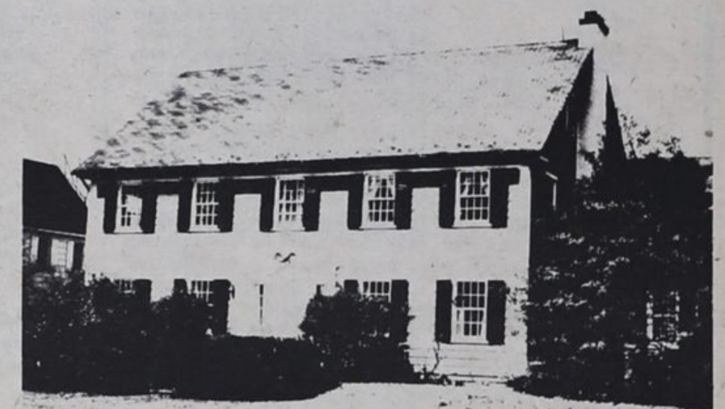
Early American Colonial with shuttered multi-paned windows, clapboard siding. Narrow vertical side-lights flank the doorway.
