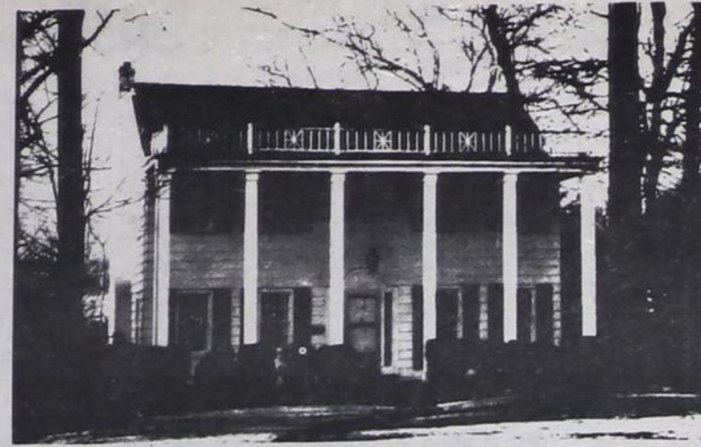
Southern Colonial in clapboard, well-scaled to lofty-columned veranda. Note the low-pitched roof with balustrade.
