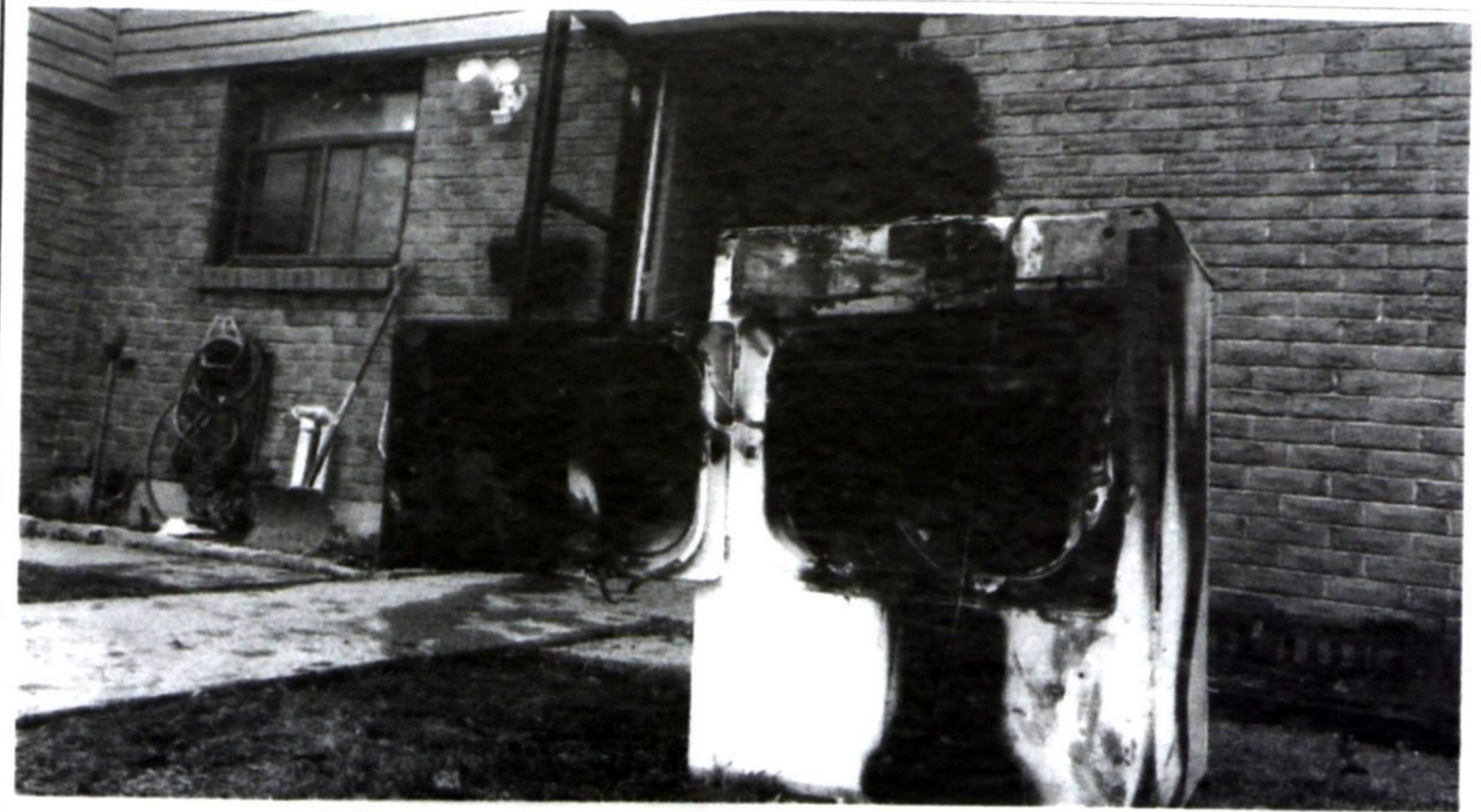
A dryer was destroyed by fire at a Commercial Street home Tuesday afternoon. Justin Greaves / Canadian Champion (Follow on Twitter @halton_photog)
