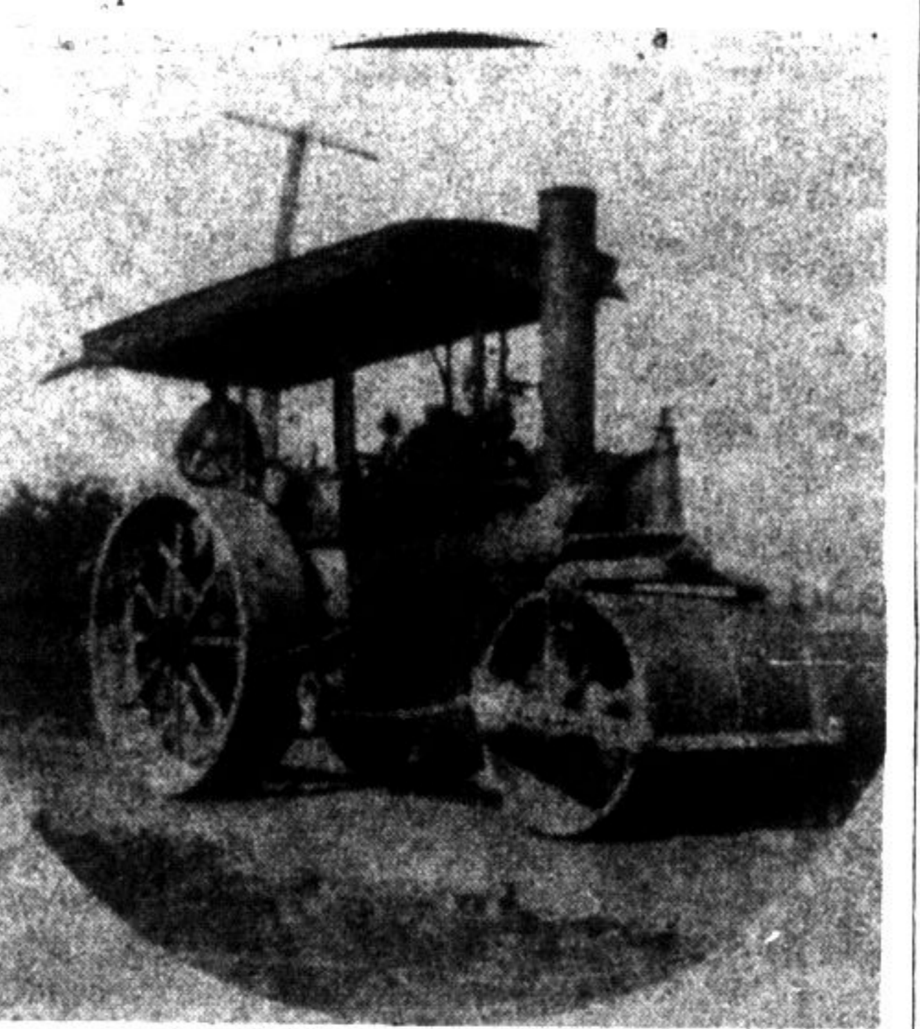
This is one of the first known steam road rollers in Halton.
