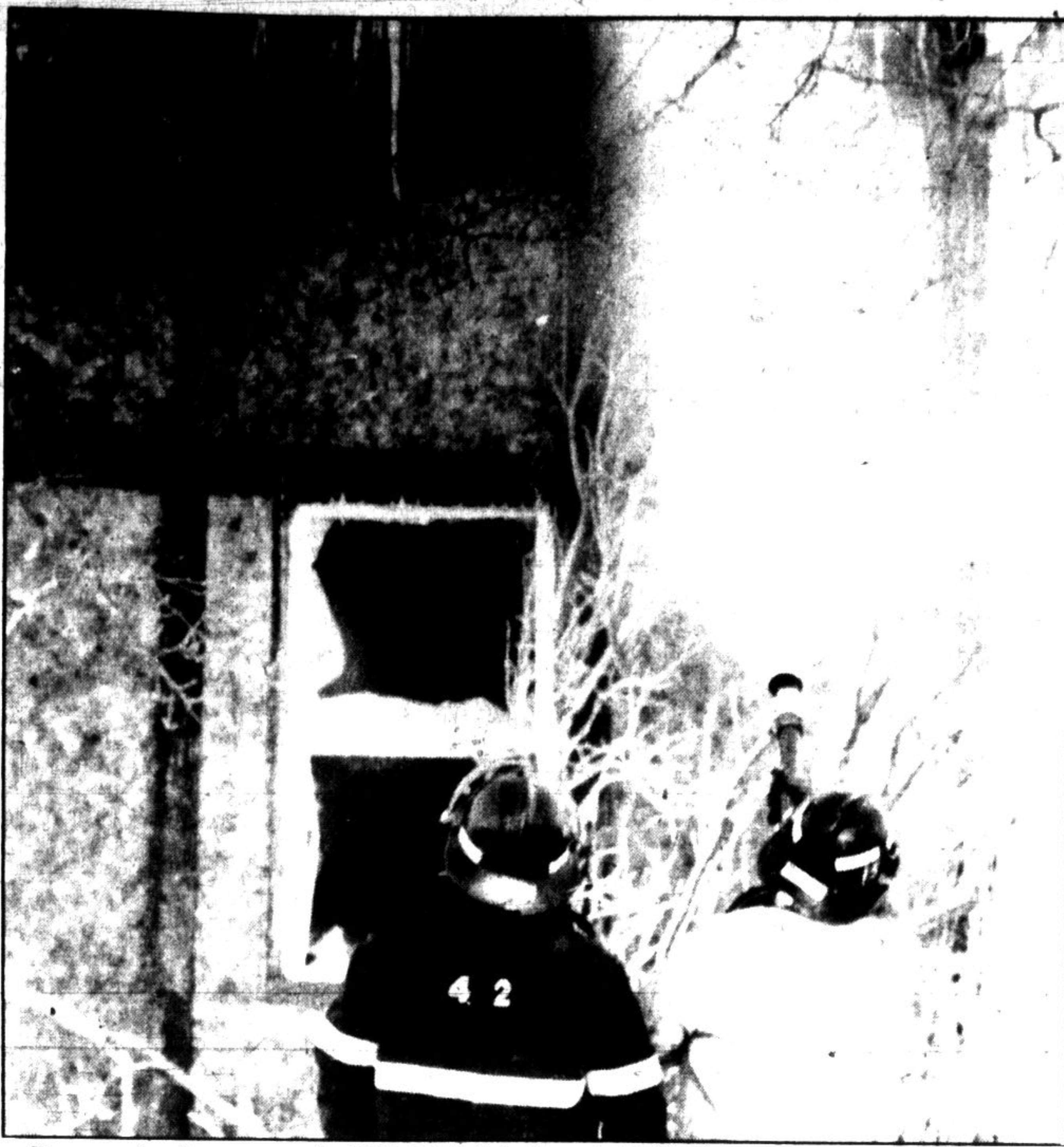
Damage has been pegged at $75,000 in this Campbellville fire. A cause has not been identified, according to Milton firefighters.
