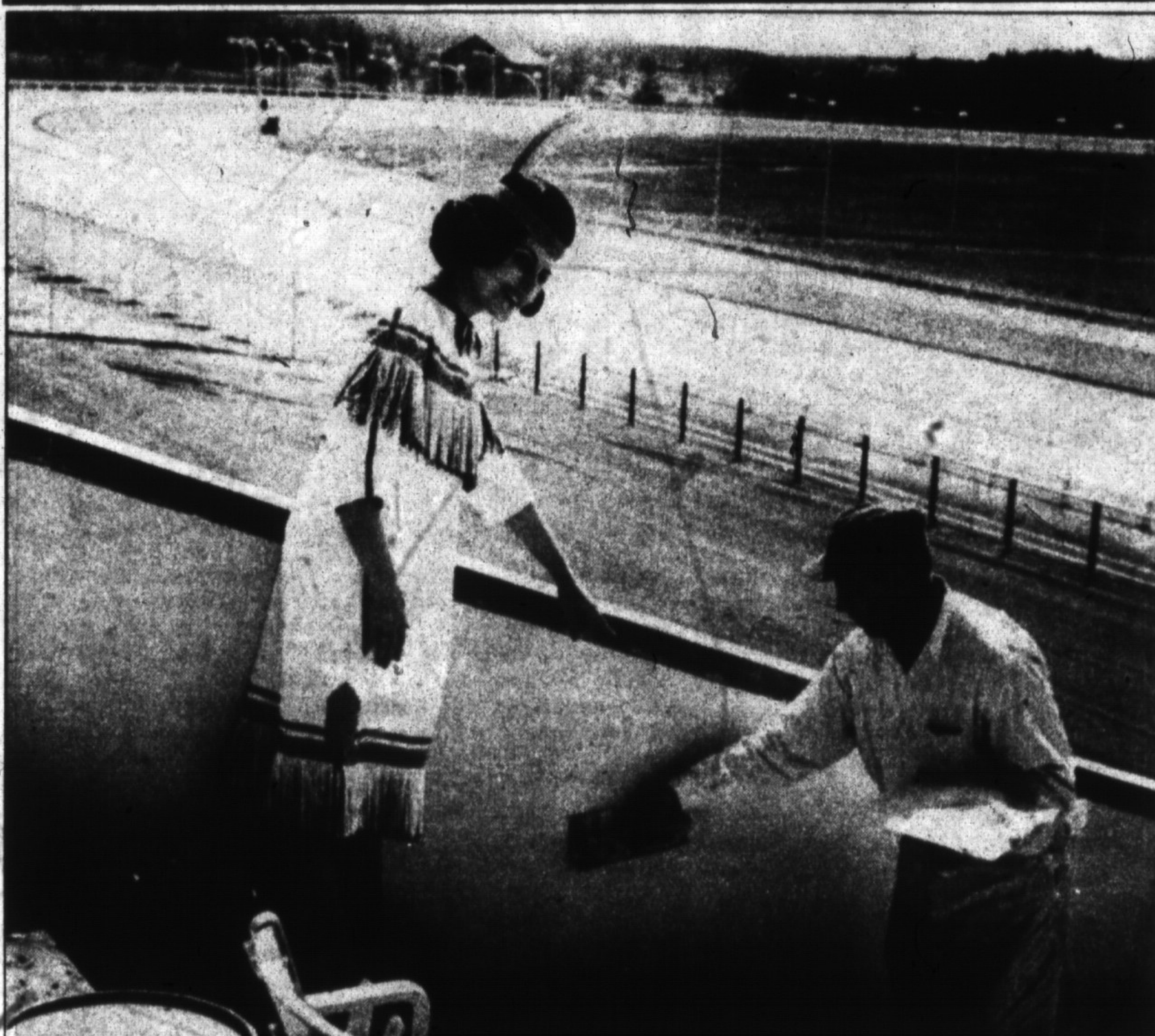
Miss Mohawk Raceway, a 25-year-old secretary, overlooks the $3 million Campbellville race track on opening day April 25, 1963. A plasterer finishes up his work on the grandstand. There were close to 100 betting windows at the track.
