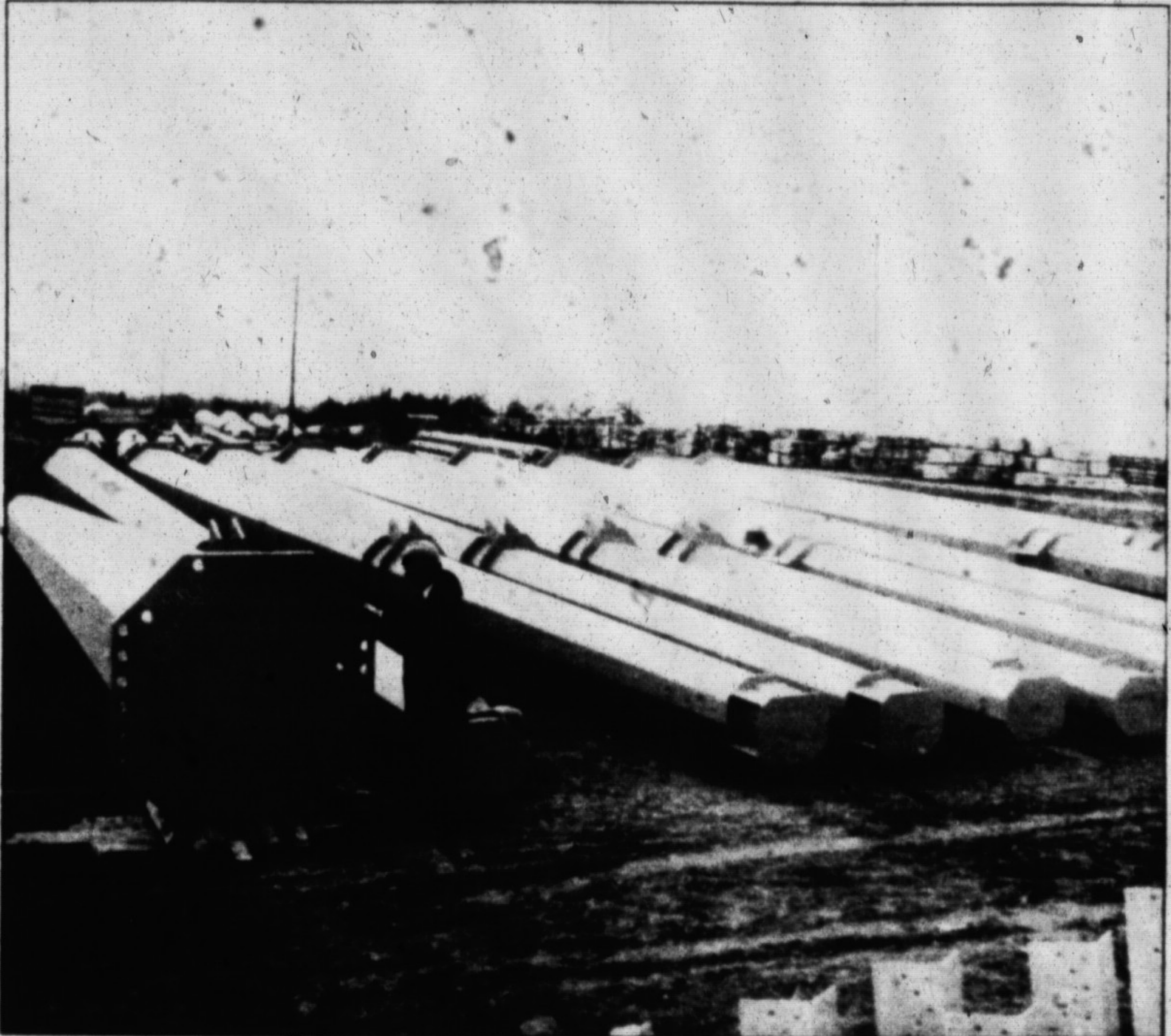
Sections of towers were being stockpiled in the Milton Hydro sjeelyard on Main Street East in November, 1976. Construction of two new hydro transformer stations was underway on Main Street East at Fifth Line and at Lower Base Line Road and Ninth Line.
