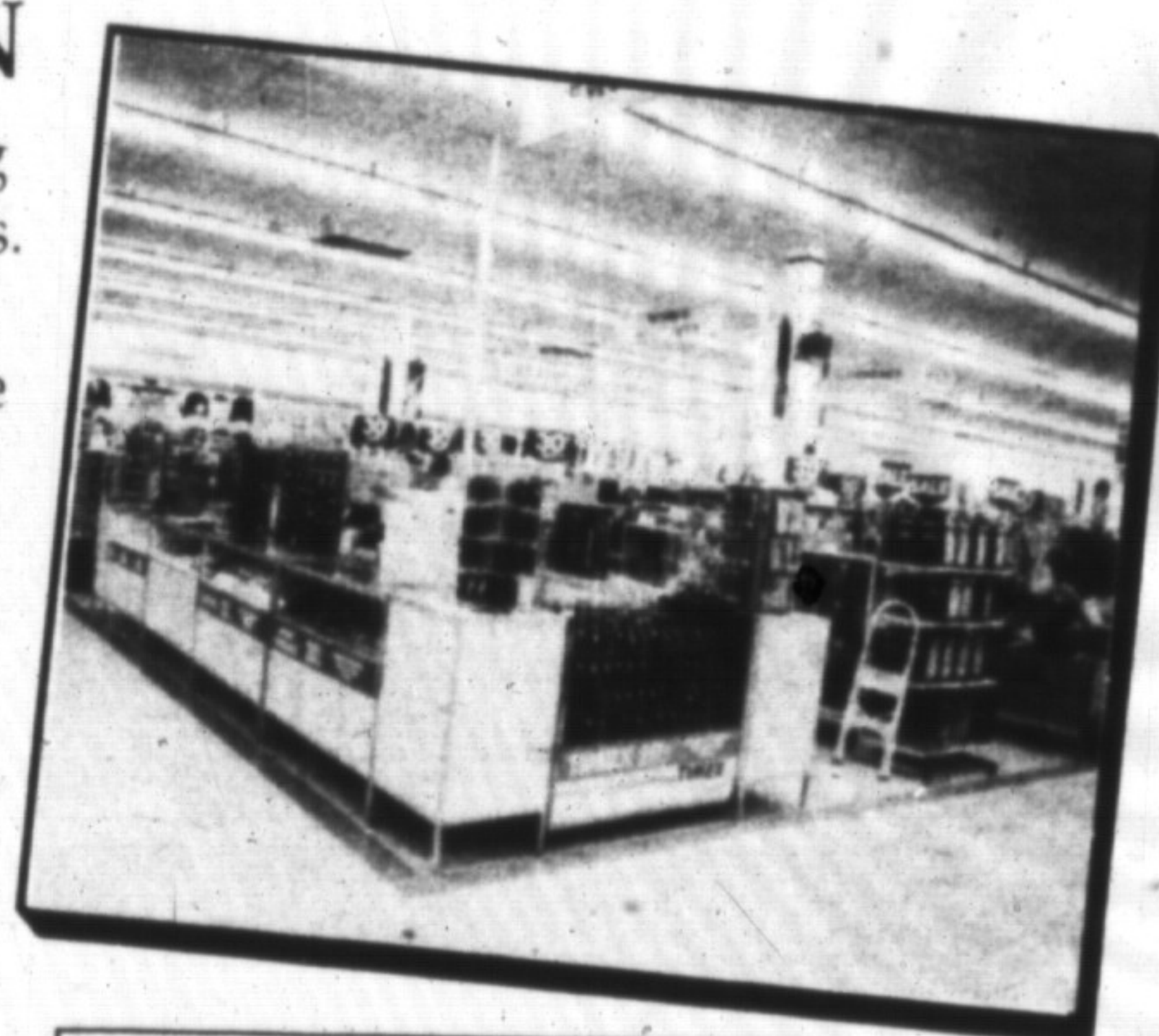
ELECTRICAL WORK DONE BY FAY'S ELECTRIC CO. LTD. 583 MAIN ST. E., MILTON
