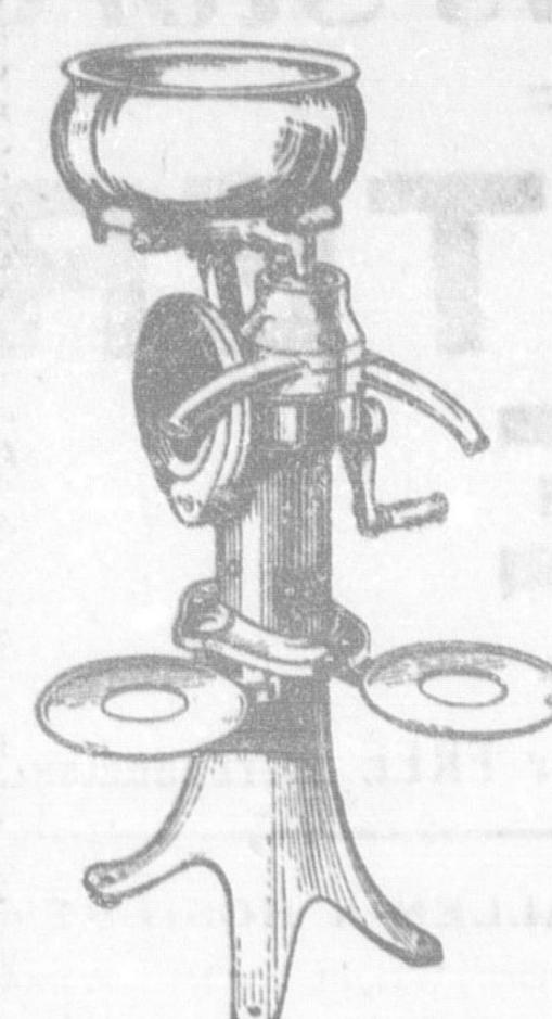
Enclosed, protected ball bearings—a friction-free spindle and the closest skimming bowl on she market make the
