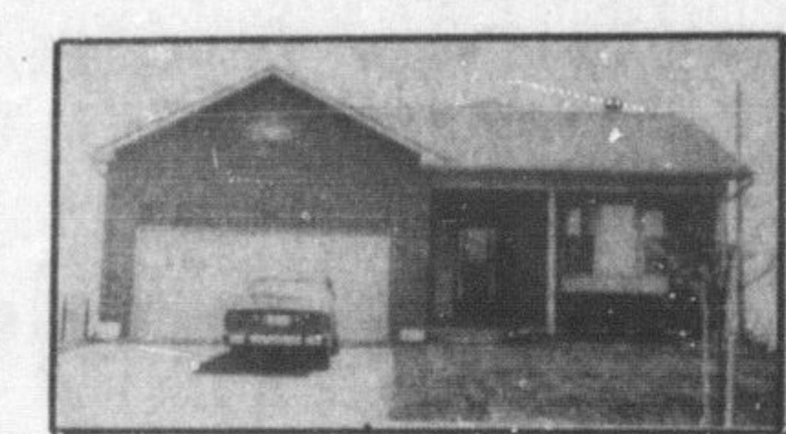
BEAUTIFUL BACKSPLIT - $129,900 4 Bedrooms, main floor family room with fireplace, lower level has finished recreation room. Double car garage. Please call Joan McCoy or Carole Stonhill.
