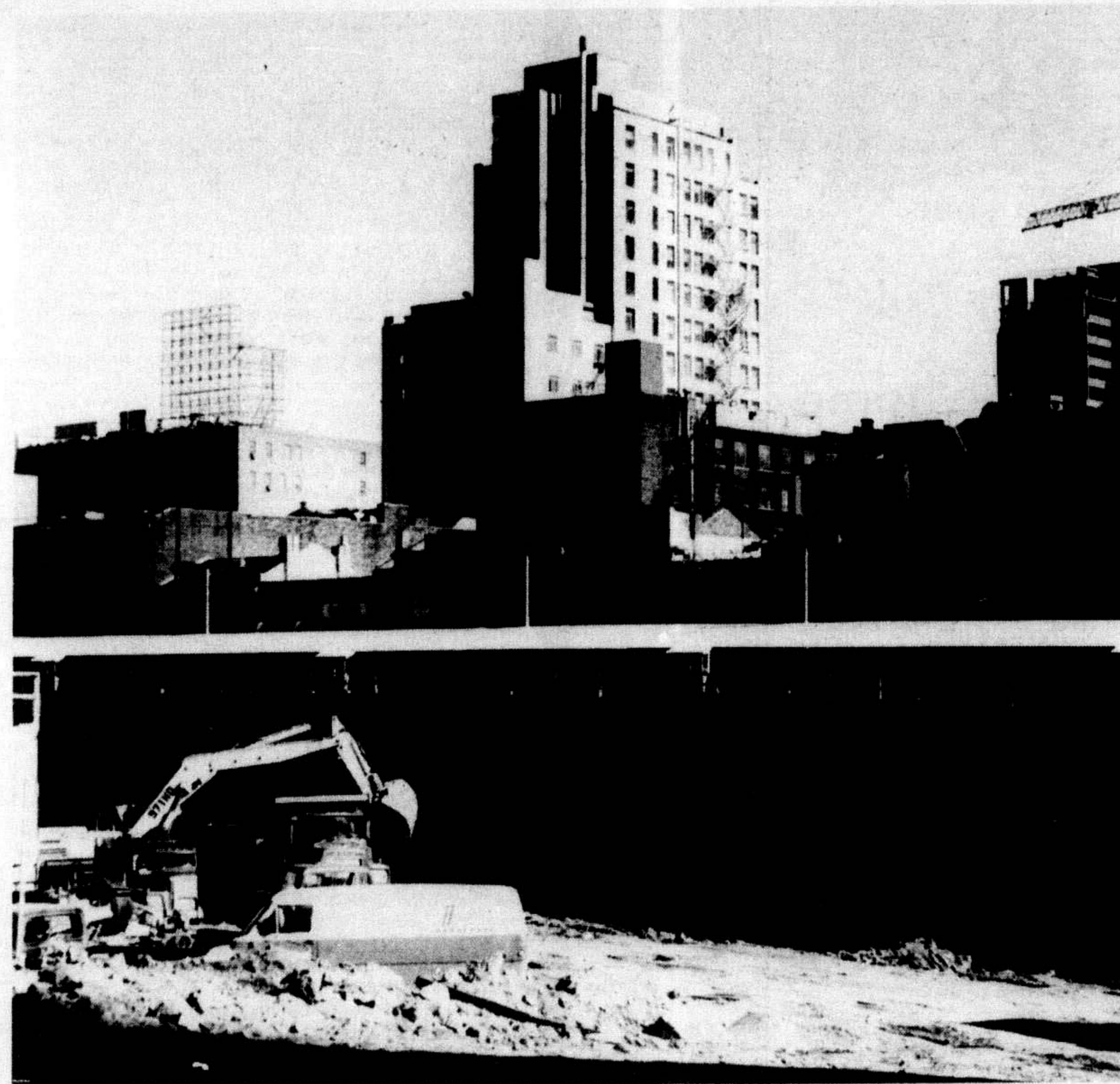
Tearing down and building up, that's the name of the game. Here the construction of the new Eaton's Centre is underway at Yonge and Dundas Streets.
