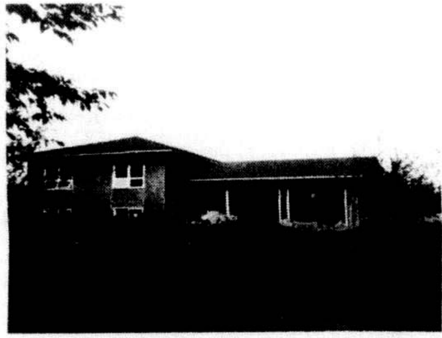
NEW 3 BEDROOM, brick, backsplit, 2 car garage. Large family room could be finished to purchaser's likes. Good country lot with a small neighbourhood of fine homes. $79,900.00.
