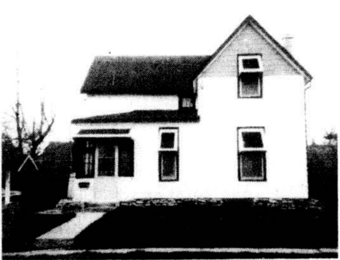
DUPLEX—aluminum siding and awnings, central location. Two 2 bedroom apartments. Large lot. One of the best buys of our time. $49,900.00.
