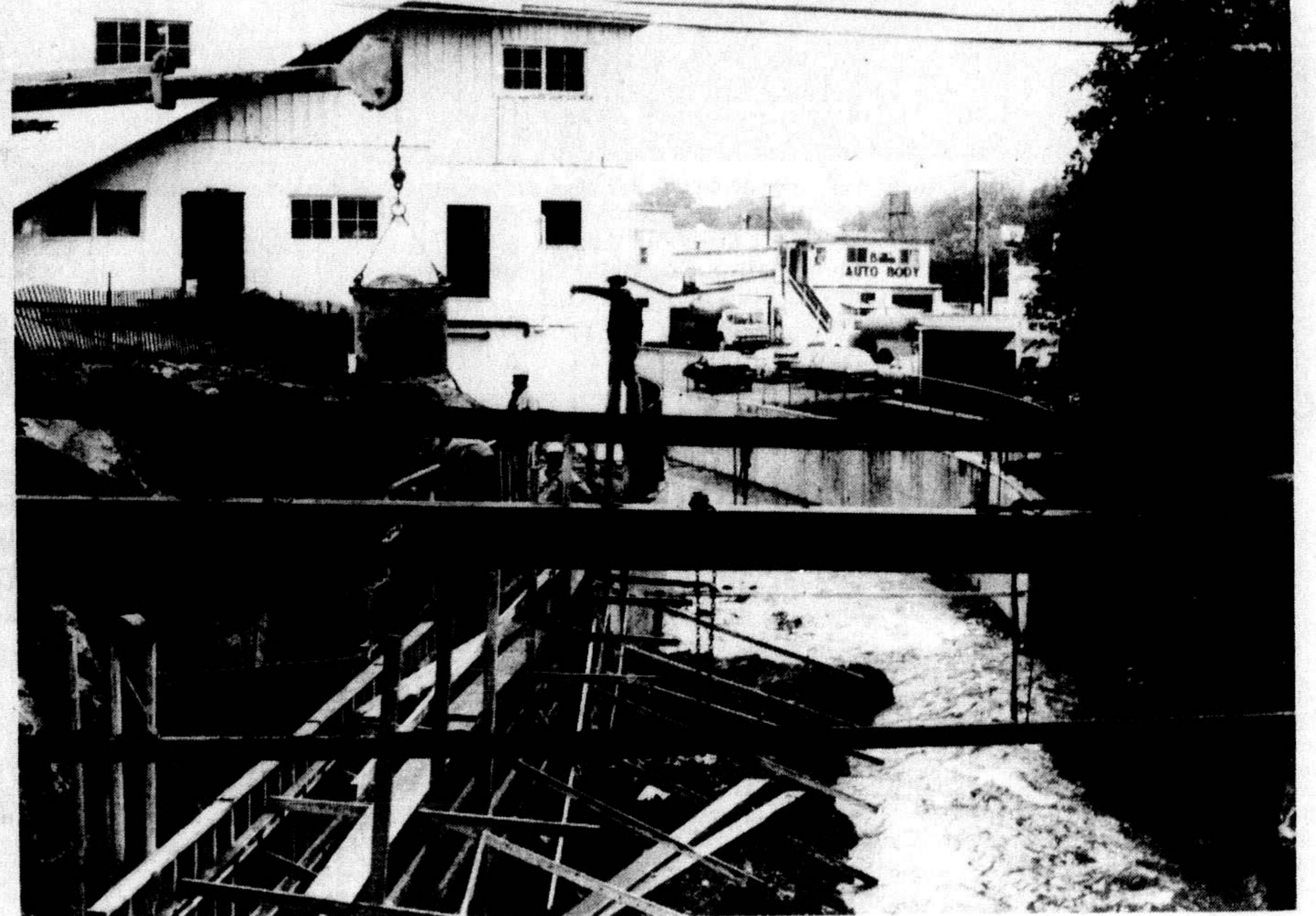
A WORKER stands gingerly on a steel beam as he directs the lowering of a bucket full of cement for a new restraining wall under construction.
