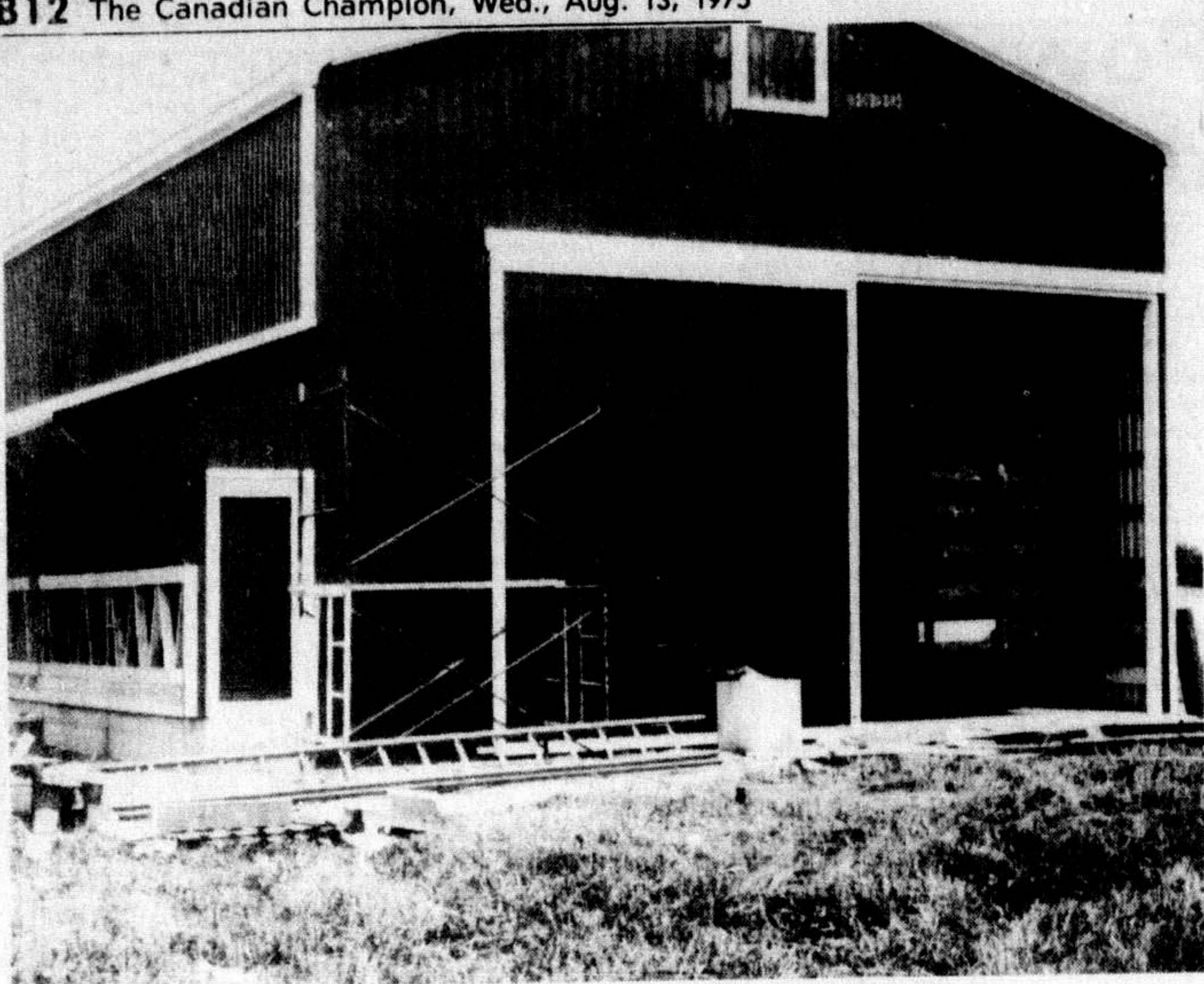
THE NEW hay barn at Valentina Farm, 15 Sideroad. Another barn similar to this one will be built later this year for housing cattle. New construction at the cattle exporting farm became necessary after a $150,000 fire razed the barn last May.
