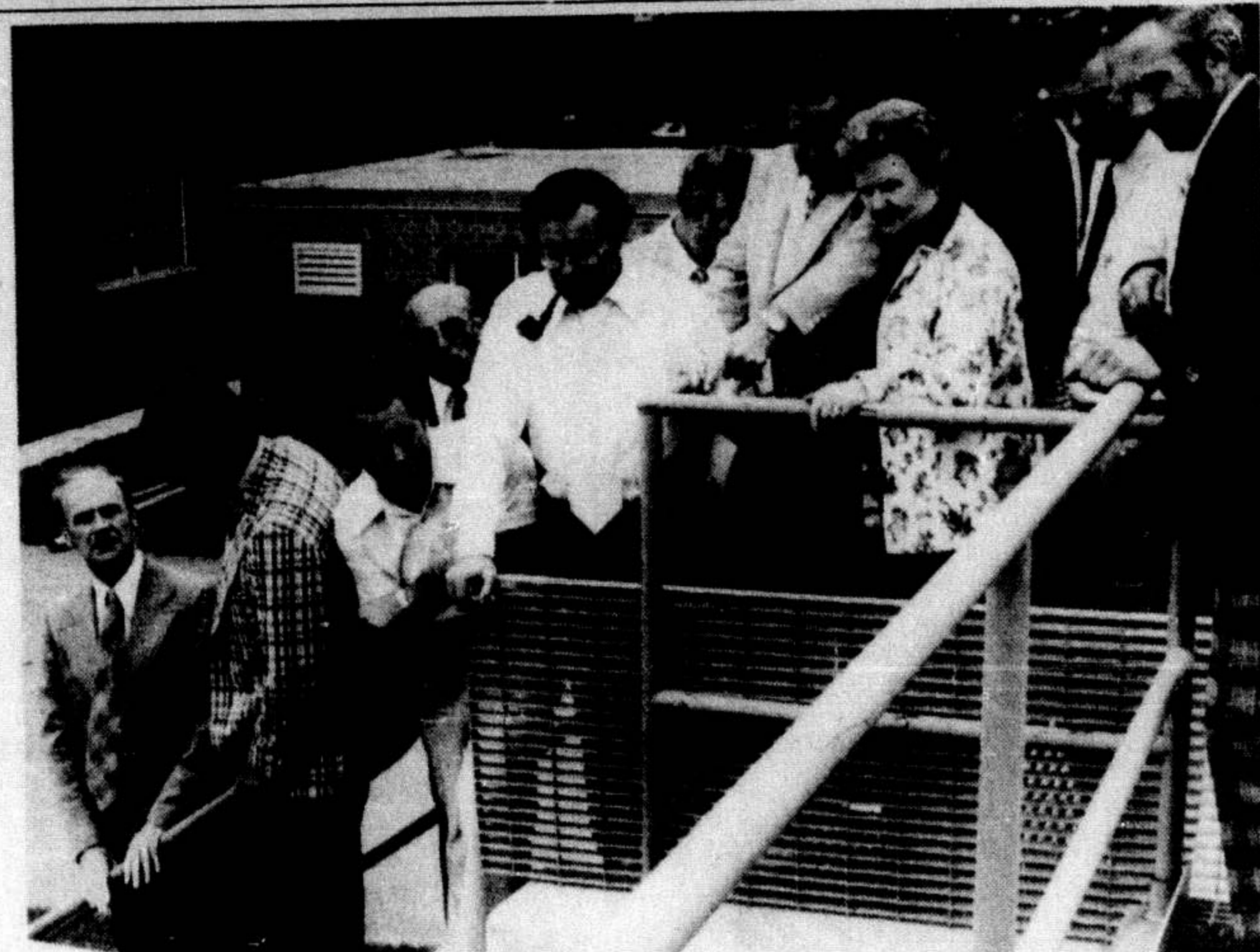
REGIONAL AND TOWN OFFICIALS took a look at Milton's Pollution Control Plant Wednesday during a tour of town and regional facilities in Milton. The town in hoping the plant can be expanded to make possible further growth.
