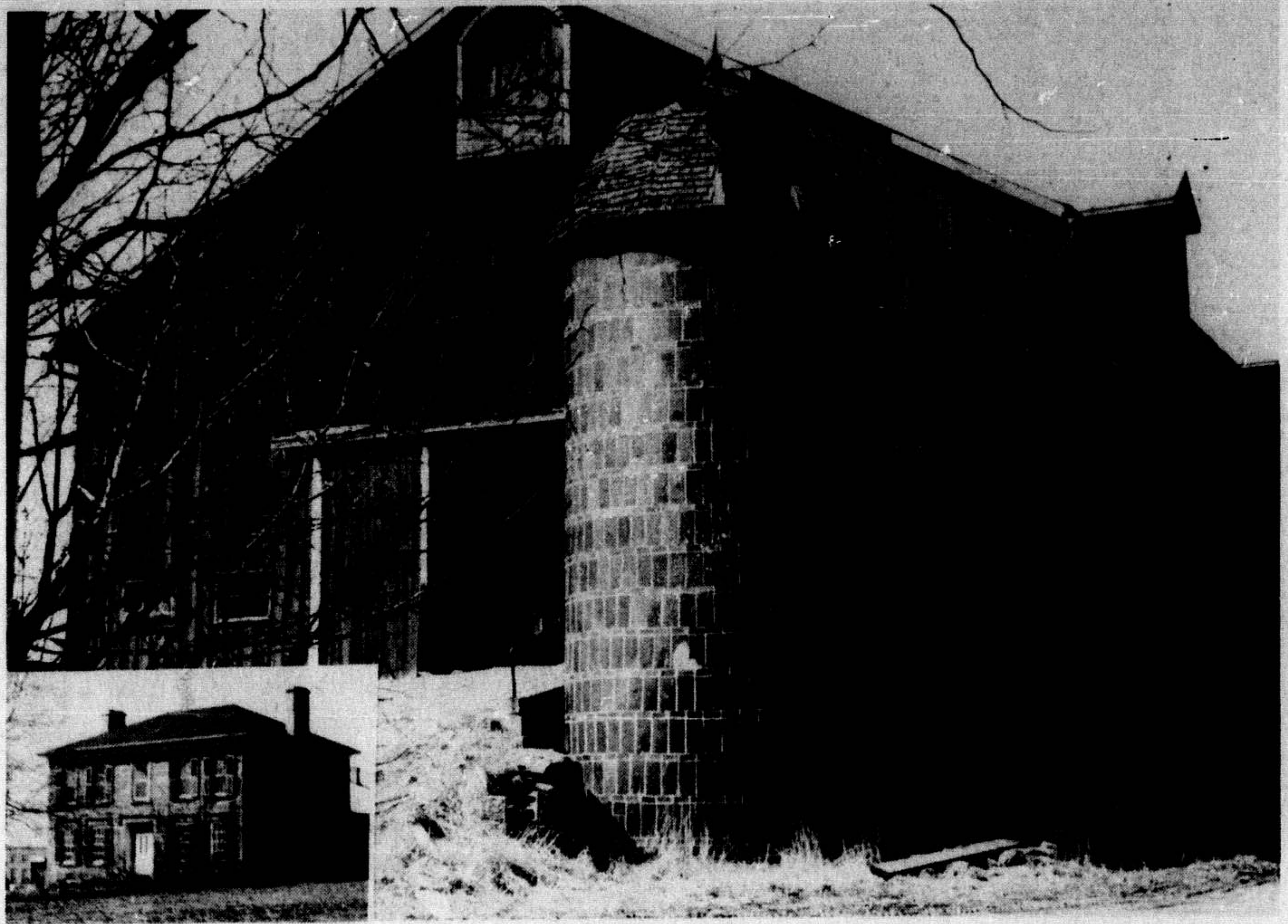
HARROP BARN is shown here before it was dismantled and carted off to the Ontario Agricultural Museum at Kelso. Built in 1882 by William Elliott, the barn is of English construction with a low pitched gable roof. It is 120 by 55 feet in size. The insert shows the stone Colonial-style house built in 1870. The Harrop family lived on the 200 acre farm for 57 years.
