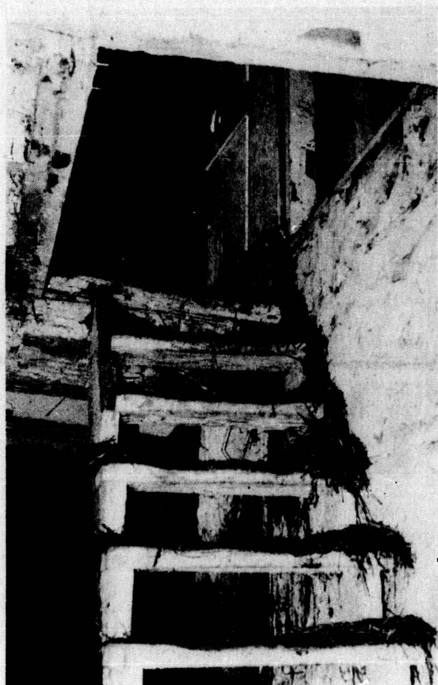
OLD STAIRS from the ground floor are well-worn. This shot shows part of the wide stone basement wall.
