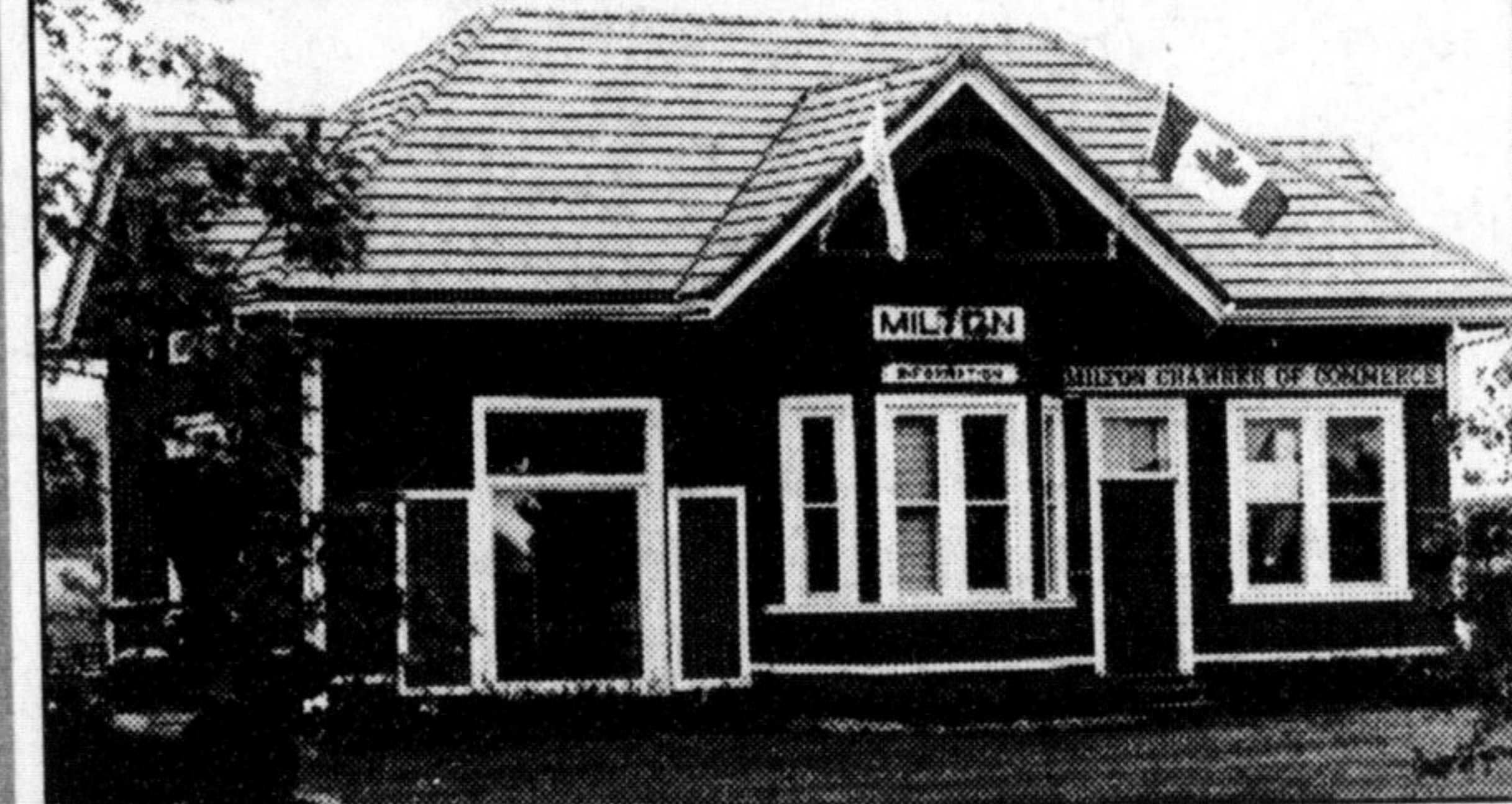
The generous donation of Marley Roof Tiles by Stirling Building Products allowed the town to maximize their capital budget allocation for a new (asphalt) roof for the Train Station in Chris Hadfield Park, home to the Milton Chamber of Commerce. The old roof had two and a half layers of shingles which took the crew over a week to remove. They then installed the new light weight Marley tiles in a few days. The colour and style of the tiles have rejuvenated the historic building and acts as a landmark for the Town.
