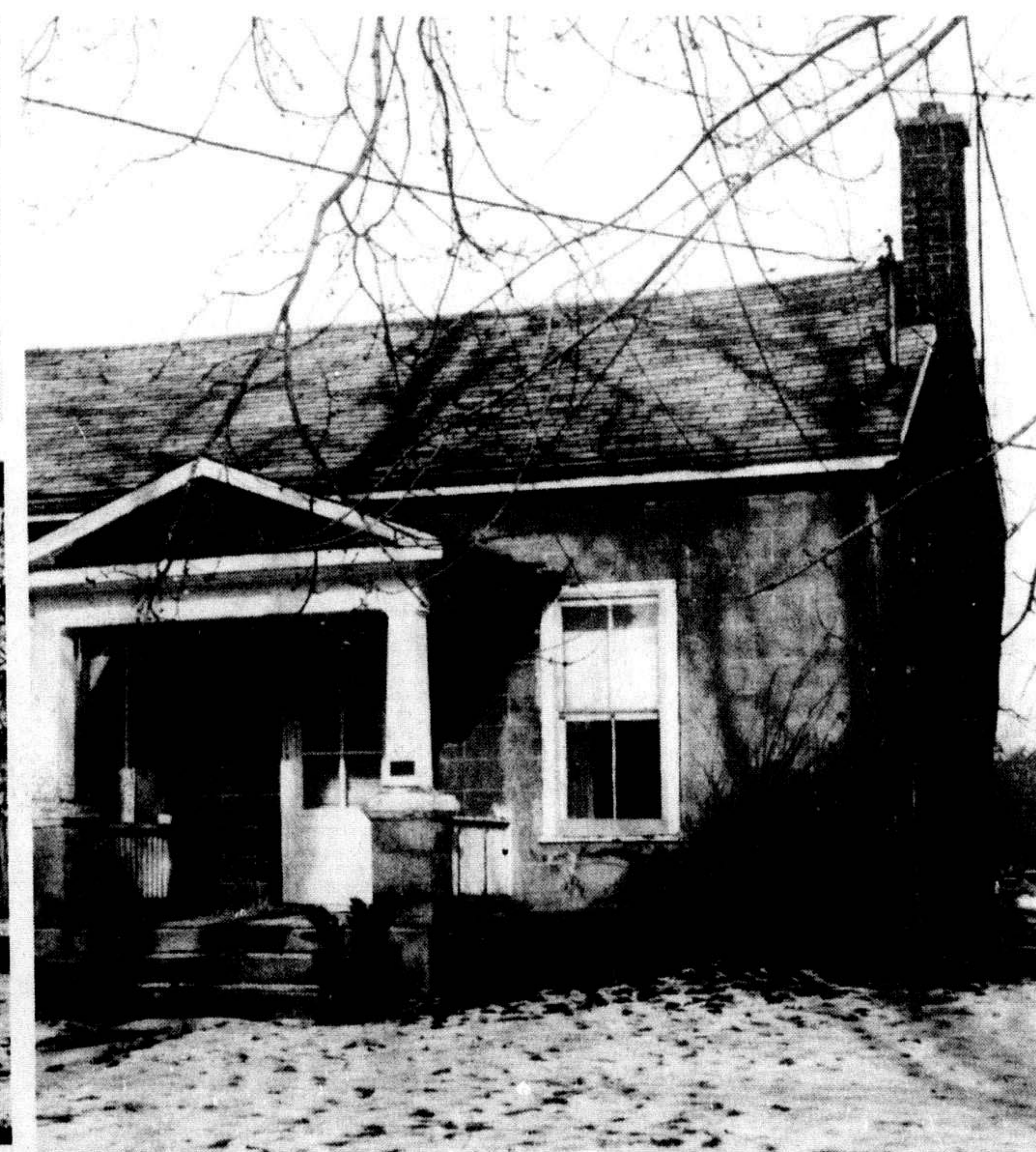
6-Original log structure of this old house is under the stone.
