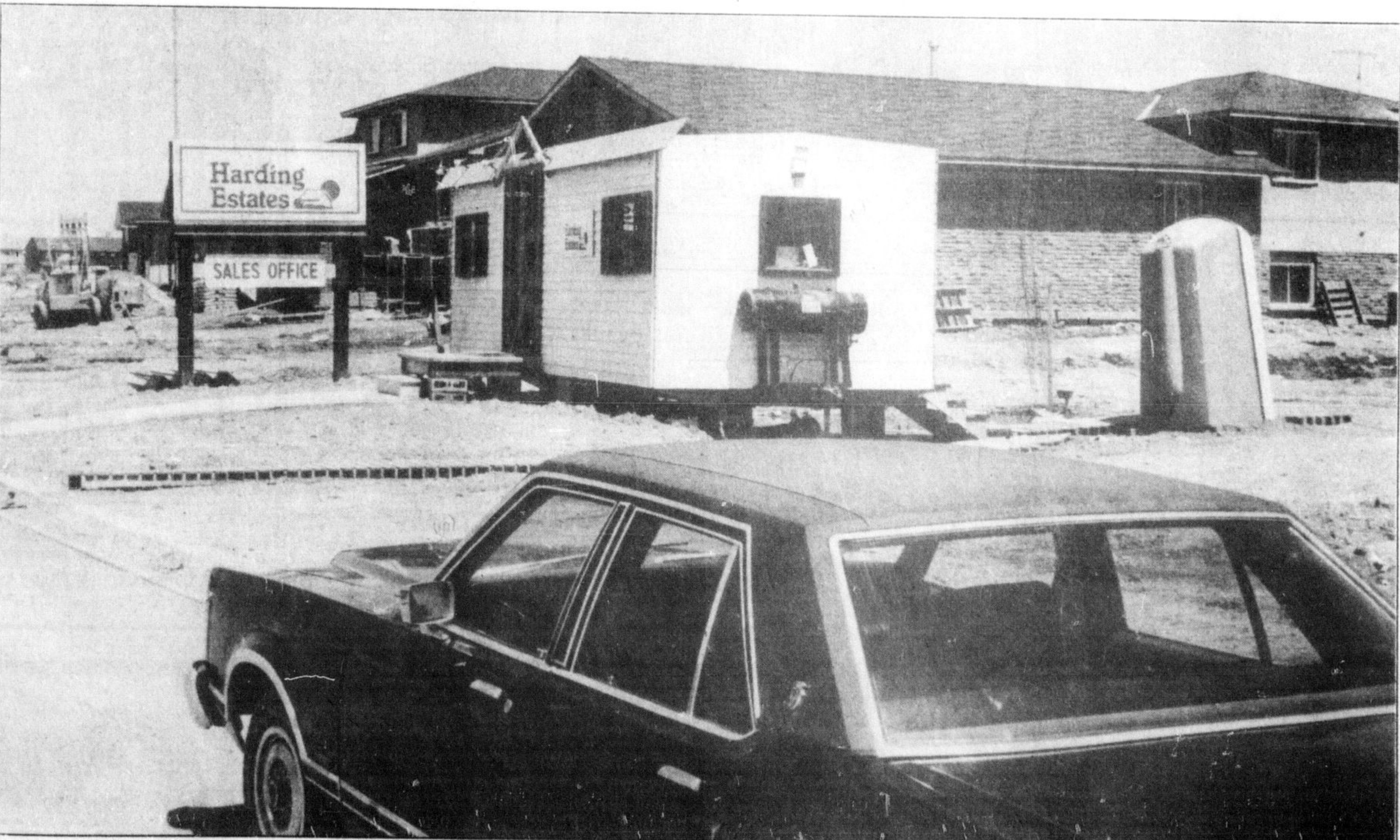
PARKED CARS , construction equipment, rows of houses, a real estate office and an outdoor toilet are characteristics of Timberlea, Milton's fastest-growing subdivision. With building permits issued for almost all of the 692 housing units in Phase One of
