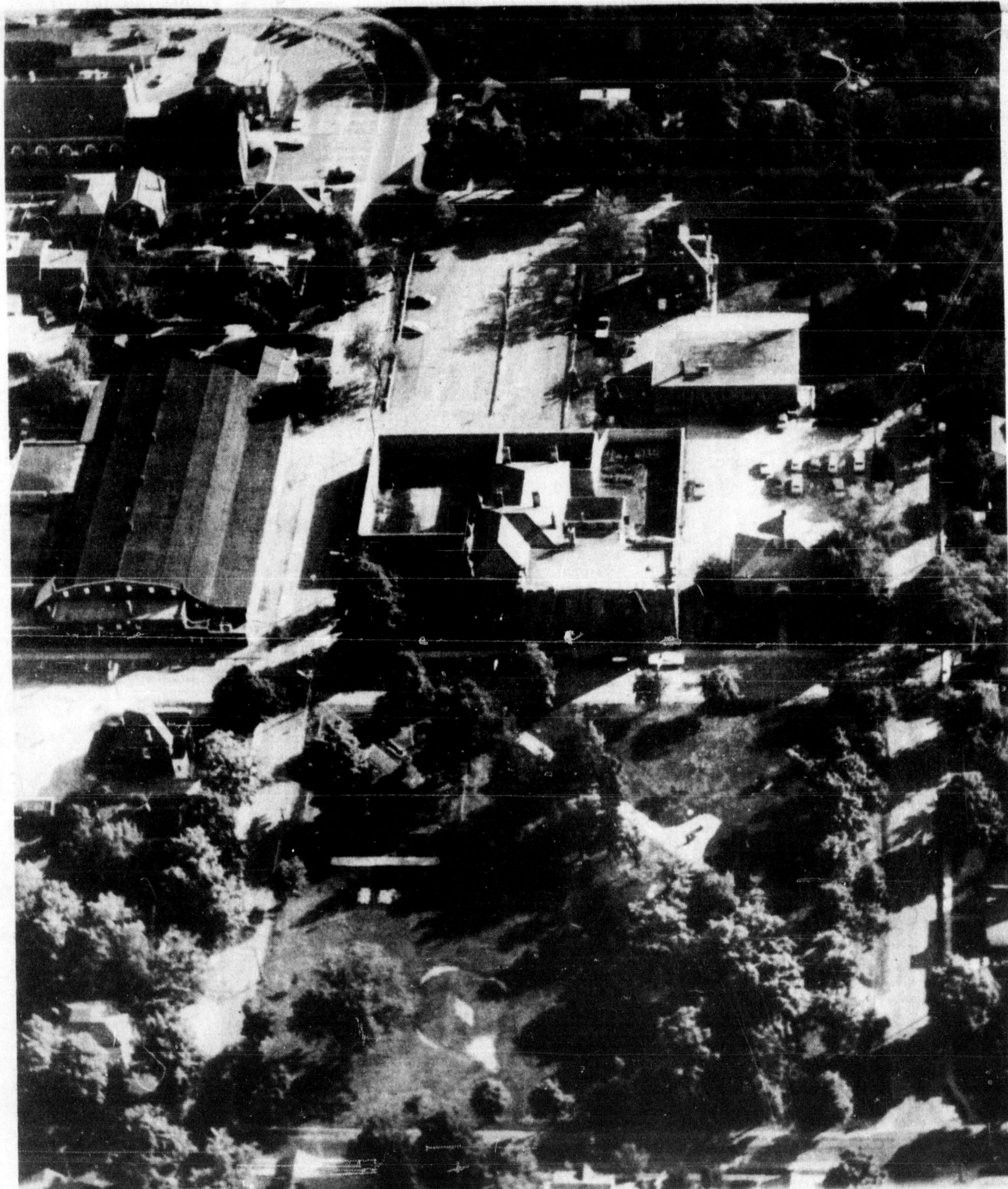
THE ORIGINAL COUNTY SQUARE, a four acre gift of Hugh Foster in 1854, is seen in this aerial view taken before the removal of the Brown St. arena. At the bottom of the photo is Bell St. with Hugh at the top. Mary St. is on the left and King St. on the right. The
