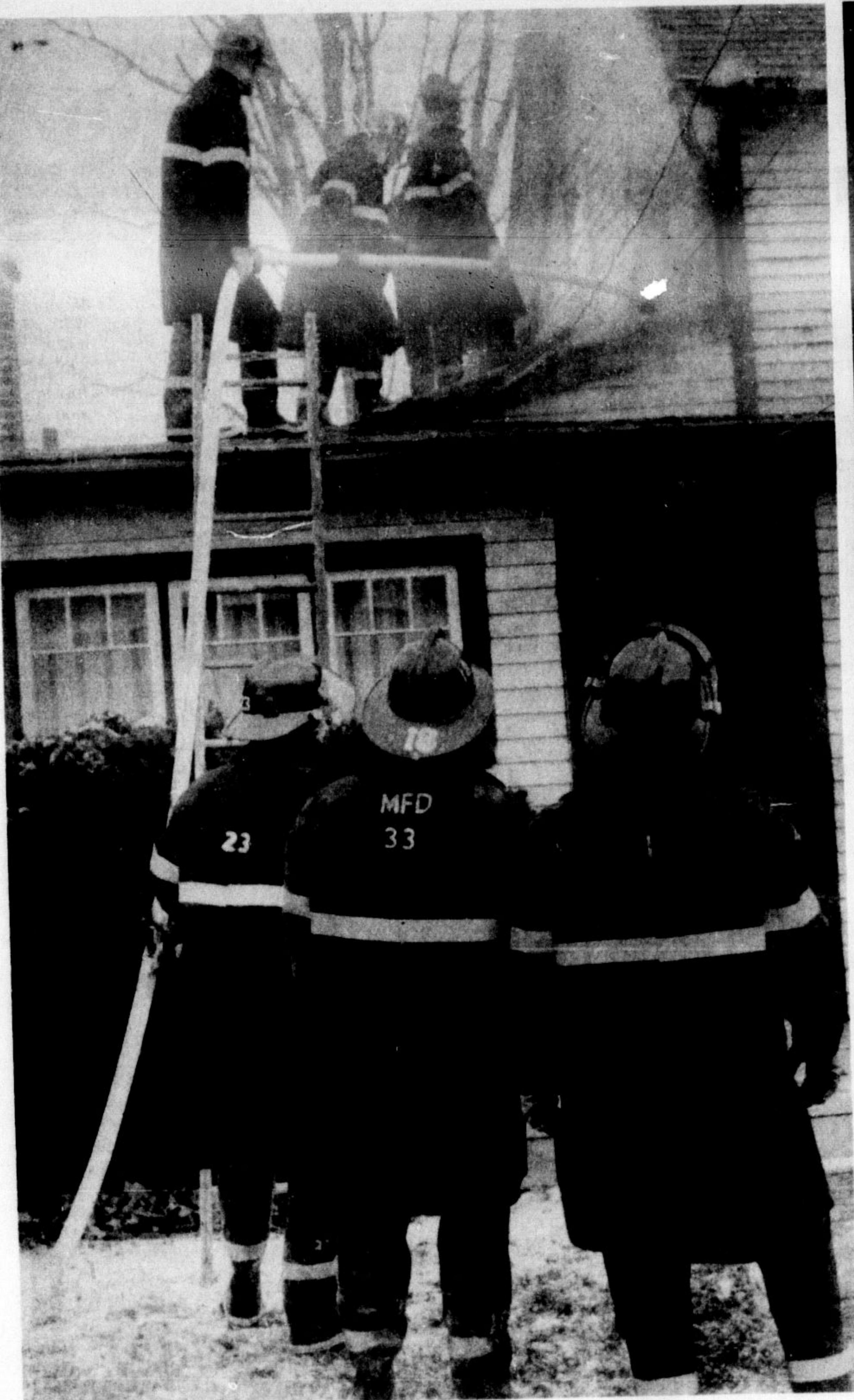
EXTENSIVE SMOKE DAMAGE was caused in a Tuesday morning fire at the home of Archie Metcalfe of 93 Hugh St. Firefighters were forced to smash a hole in the wall to douse the fire which spread from a downstairs shed through a wall into the upper floor of the house.
