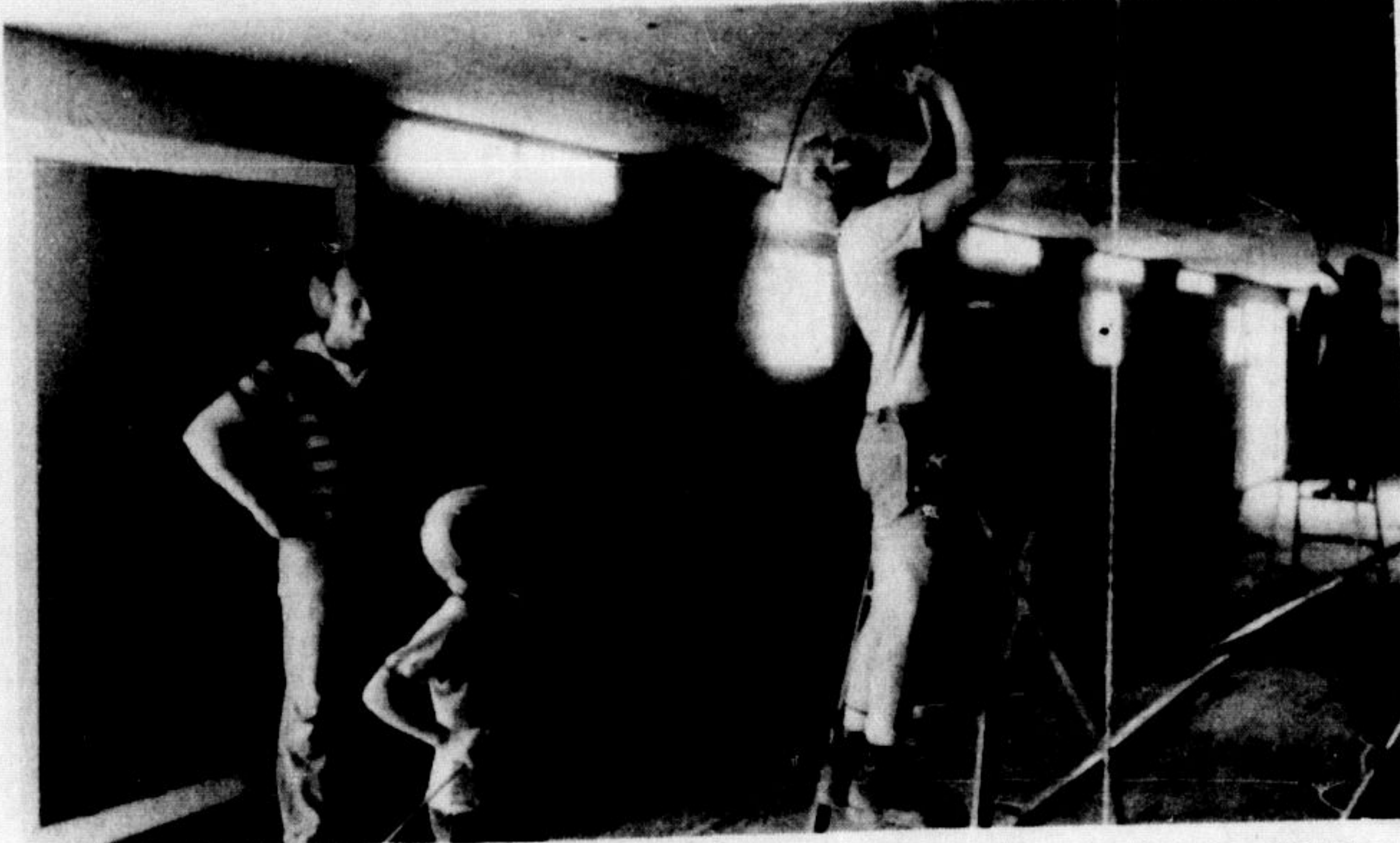
COMPLETING the lighting wiring for a new barn to house 23,000 chickens are Ed Martin, on ladder, and his young helper, nephew Jasper Martin, 8. Supervising the operations is owner Charles Martin. The chicken operation will now supply approximately 200,000 broiler chickens annually to area grocery warehouses.
