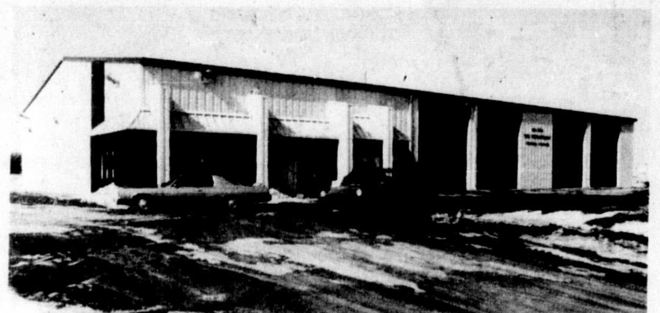
Milton Fire Department last week moved into its new home, the new steel fire hall building on Steeles Avenue. The building was purchased by Milton Council last year and erected by Transway Steel Buildings, at an approximate cost of $400,000. Congratulations to the firefighters on their new quarters.
