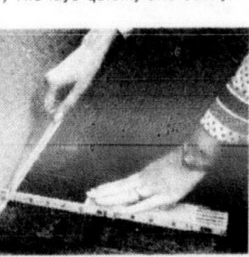
(9) Don't bind the flooring against the side walls. Leave a 1/2-inch expansion border Cover the void with the base
