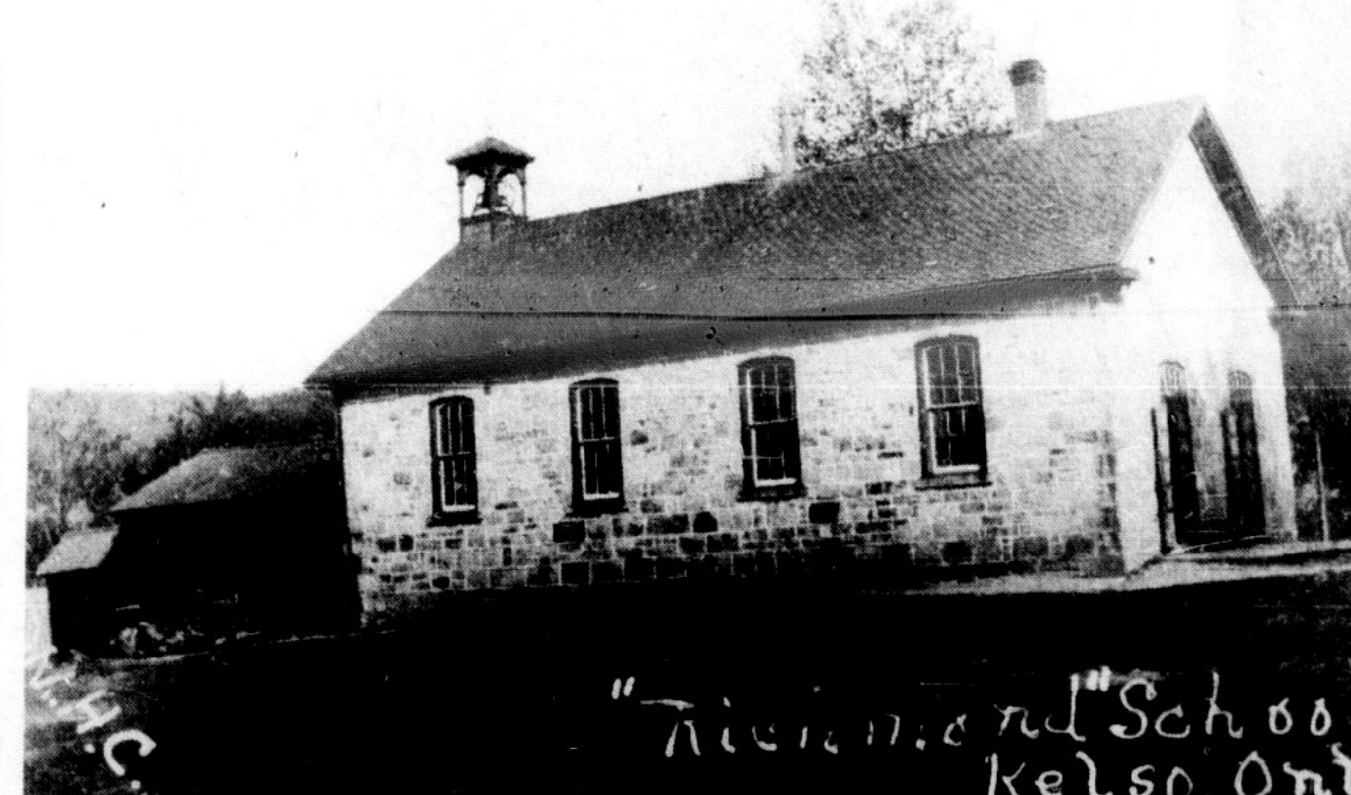
THE OLD RICHMOND SCHOOL at Kelso is in the news again. Council has invited interested groups to submit proposals for its preservation and use. The photo is from an early postcard, loaned by Larry Phillips of Milton. The outdoor "facilities" have been removed since this photo was taken—and someone has stolen the school bell, too.
