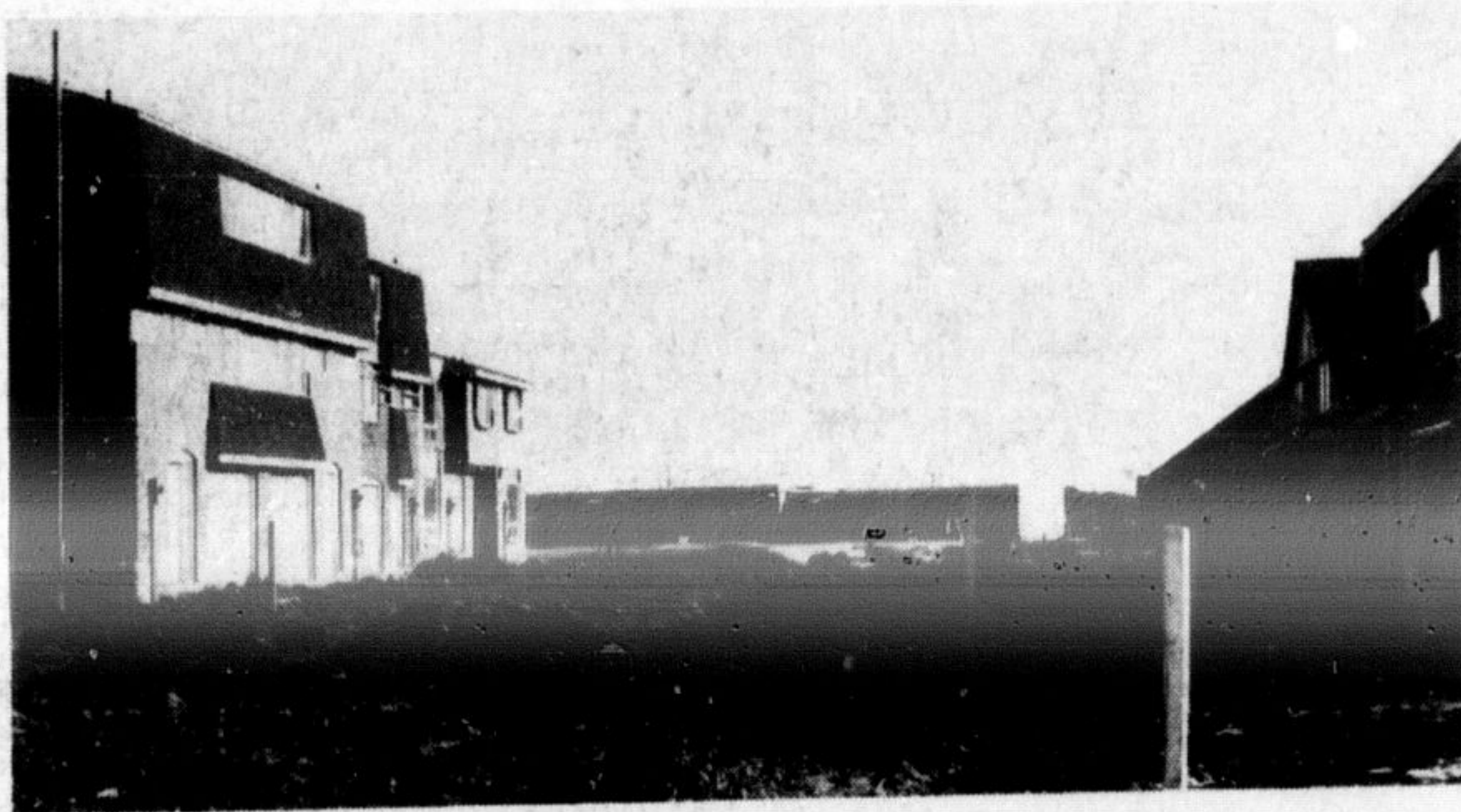
Construction began recently on 70 townhouse units in the Valleyview Subdivision on Ontario St. The homes are being built by Westbury Development Ltd. The townhouse development is one of several to be built in Milton in the past year. The town house development adjoins a single family area in the same section.
