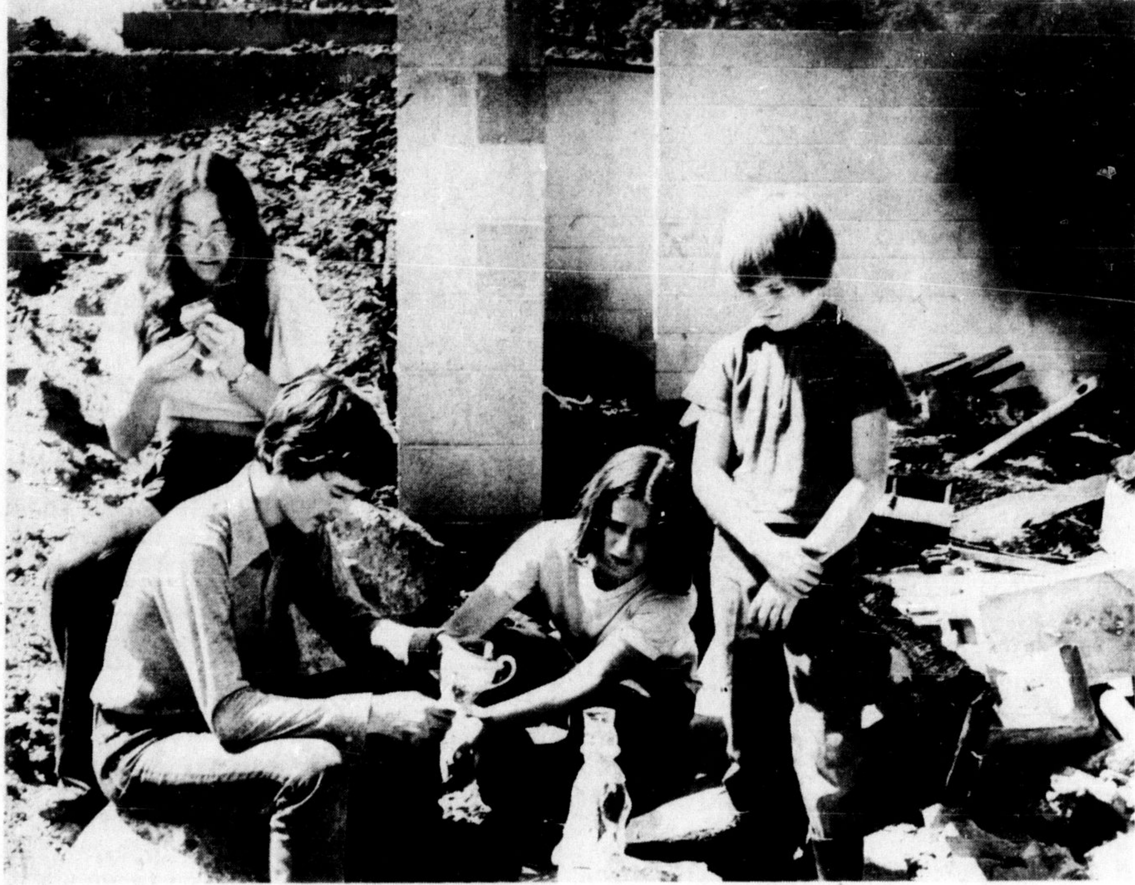
SIFTING THROUGH THE RUINS of their new home, destroyed by fire Monday night, are Sharlene and Bruce McKenzie and neighbors Susan and Barry Pickett, with whom they have been staying since the fire. They recovered some of the silverware and ornaments in the ruins of the fire Tuesday morning.
