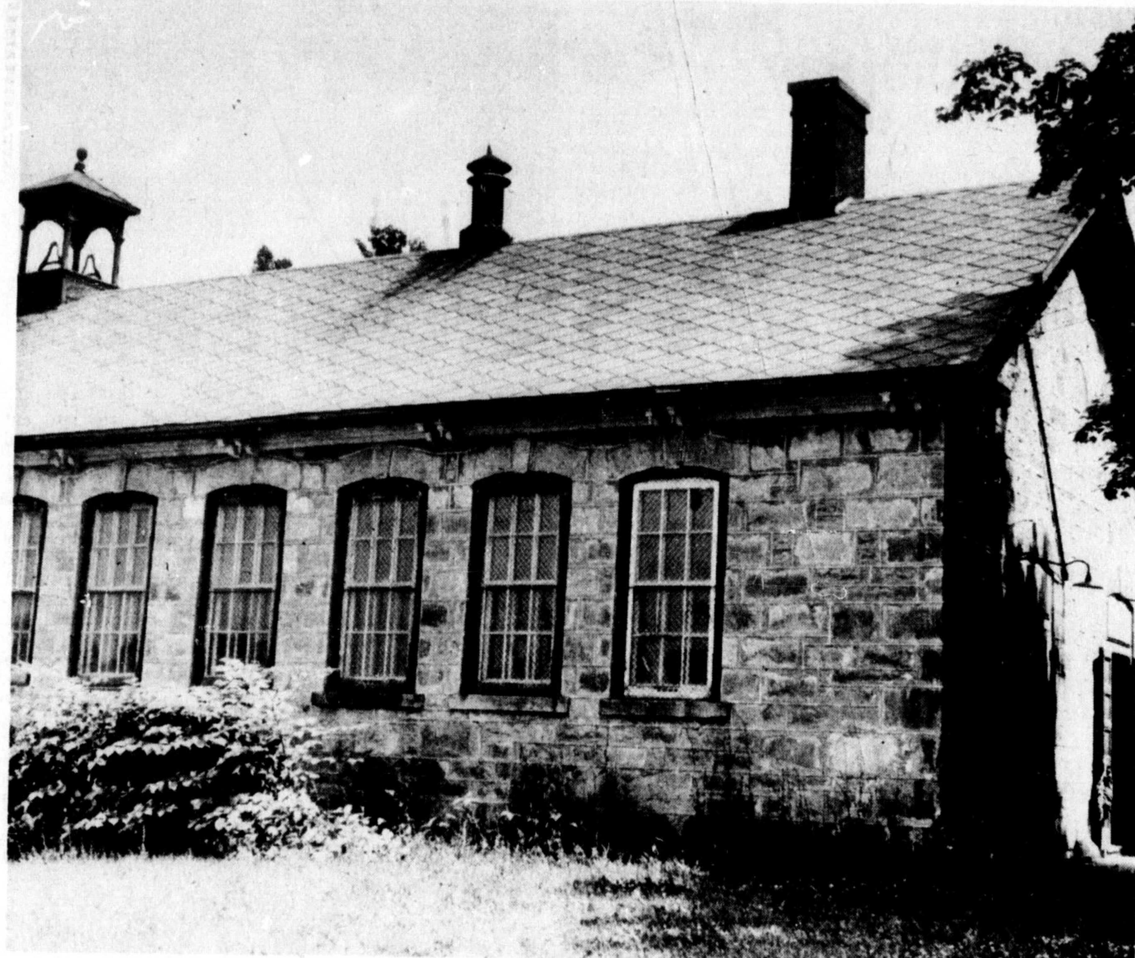
RICHMOND SCHOOL, alias Christie, alias Kelso, better known as No. 6 is a one-room structure located on Appleby Line, south of Highway 401. It began as a frame building in 1863 and the present stone structure was built in 1886. It was closed in 1965. The future use and ownership of the school is presently the subject of political bantering.
