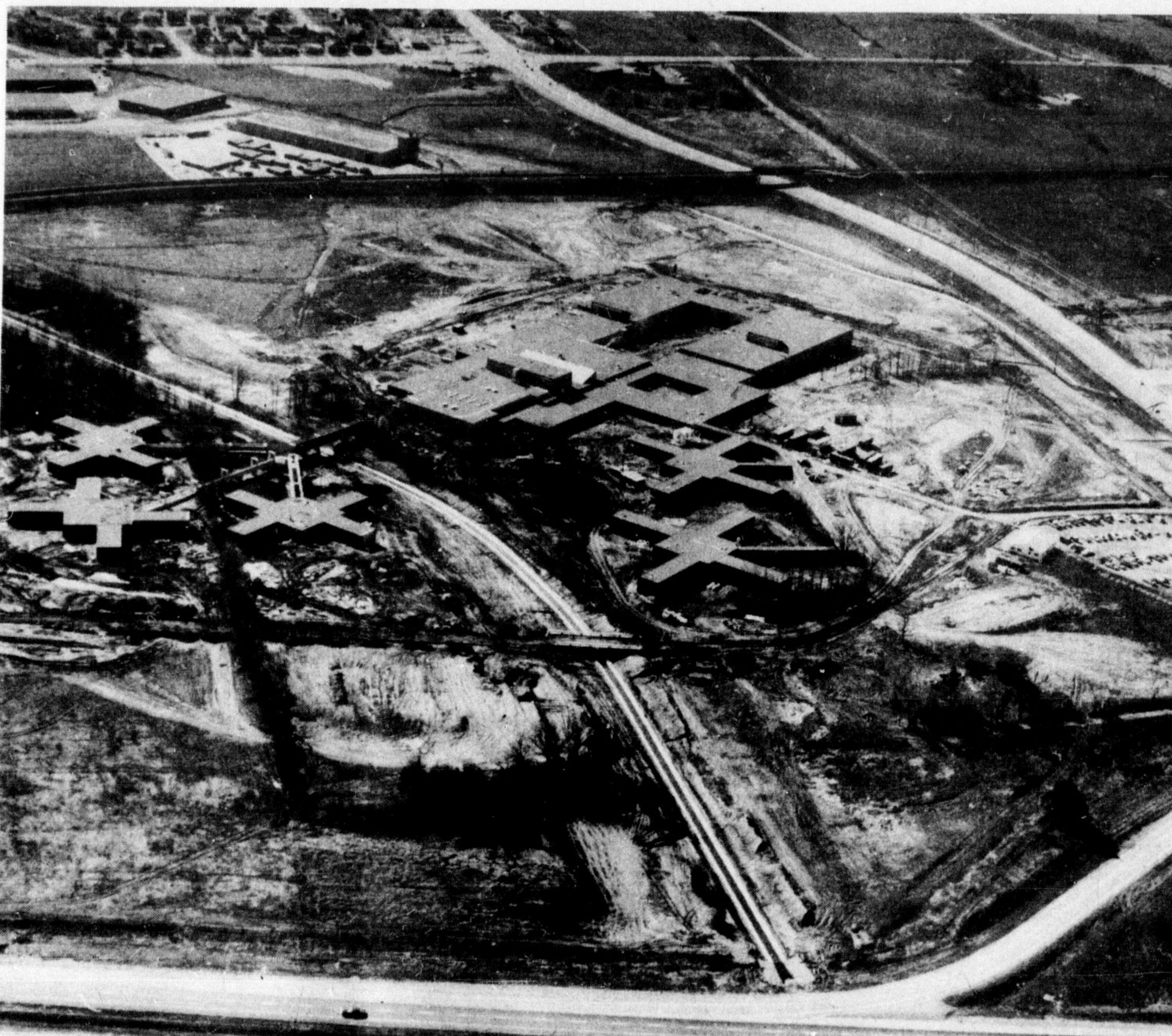
MAPLEHURST CORRECTIONAL CENTRE IS nearing completion. The $13,500,000 ultra modern facility is scheduled to be completed by March. The aerial picture gives an accurate view of the sprawling complex.
