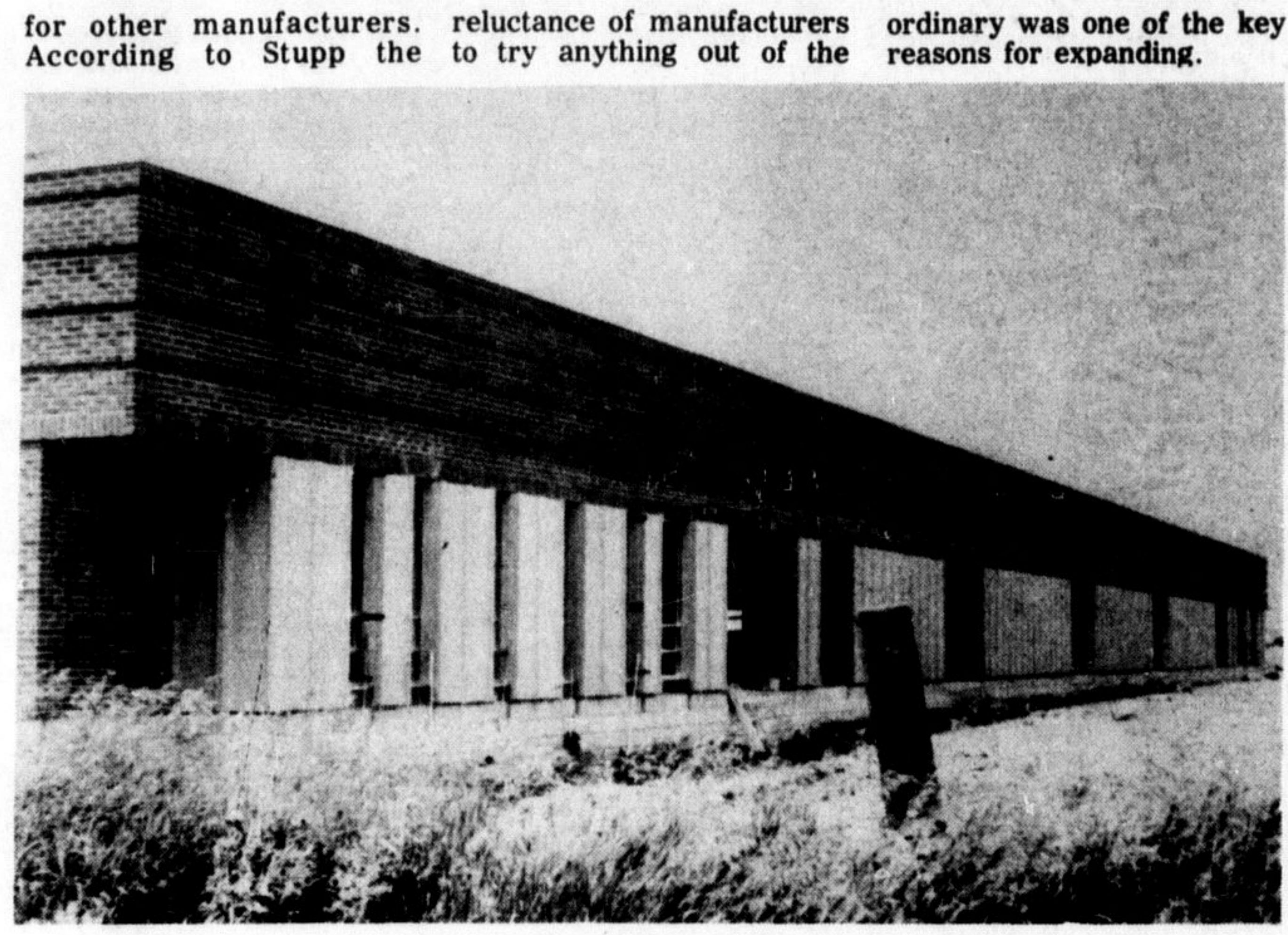
GOLDEN TRIANGLE FASTENERS hopes to be in production in August at their Harrop Dr. plant. The 29,000 square foot plant makes provision for sauna baths, showers and a pool room for employees. A demonstration of new techniques in the business was held there Monday for the benefit of representatives of the trade media and local press.
