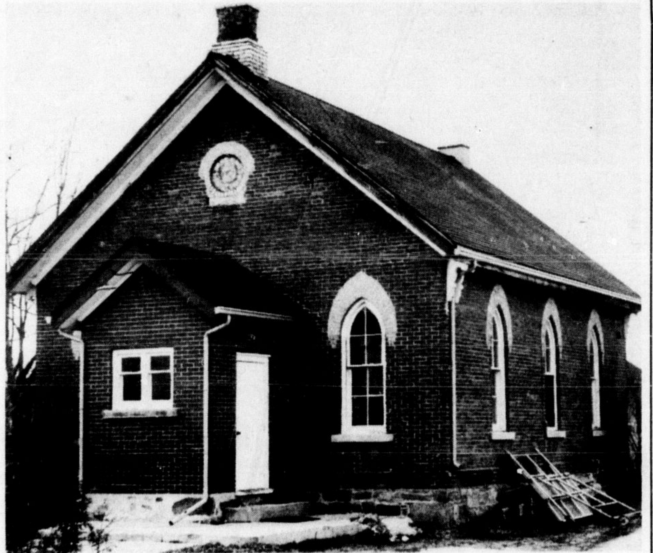
The Lorn school S.S. No. 12 erected in July 1882 is situated just north of Acton on highway 25.
