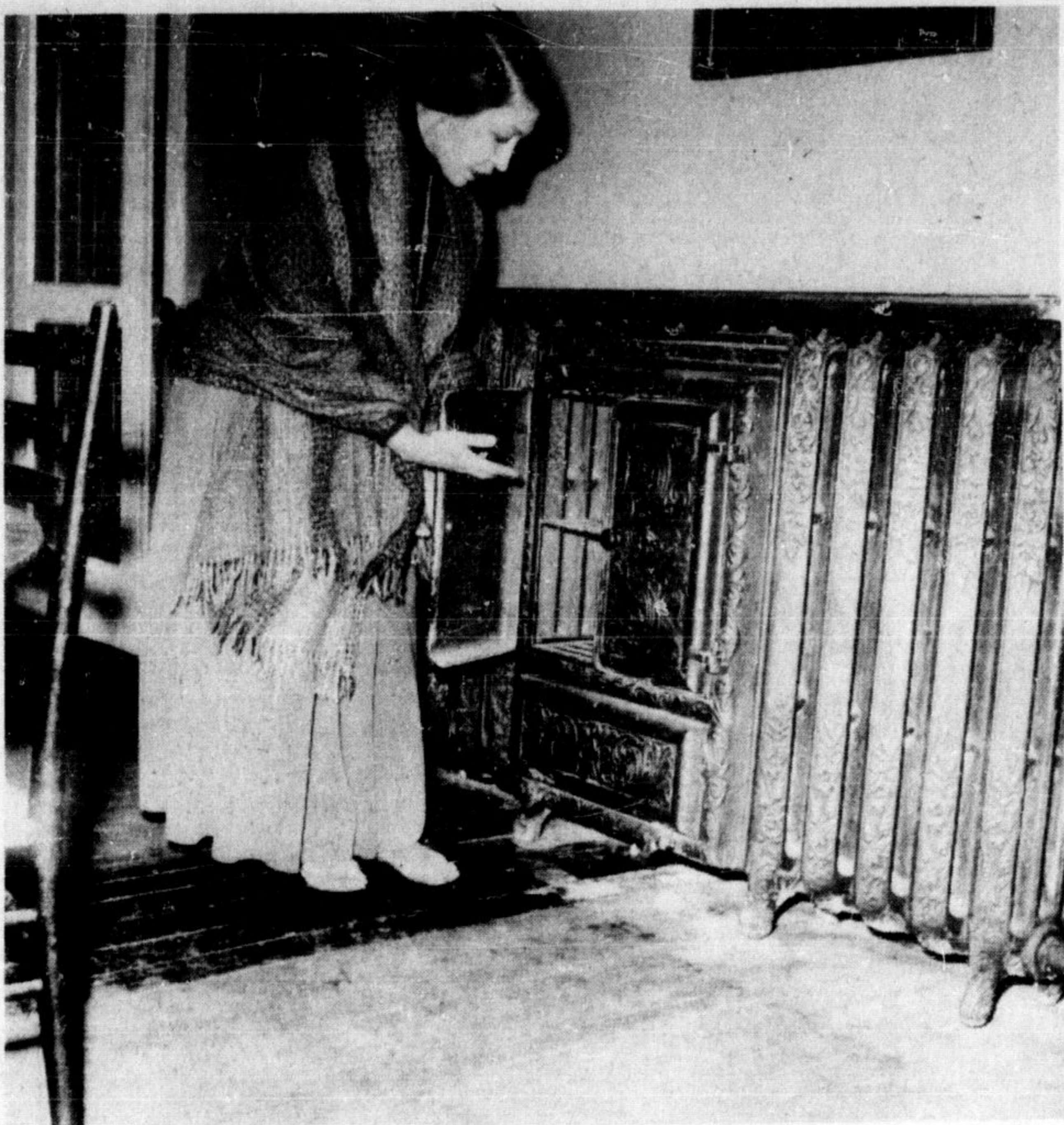
STOVE-LIKE COVER on the hot water radiator in the old Crawford house is just one of its interesting features. The Beswick household uses the "oven" to warm mitts and boots in winter.
