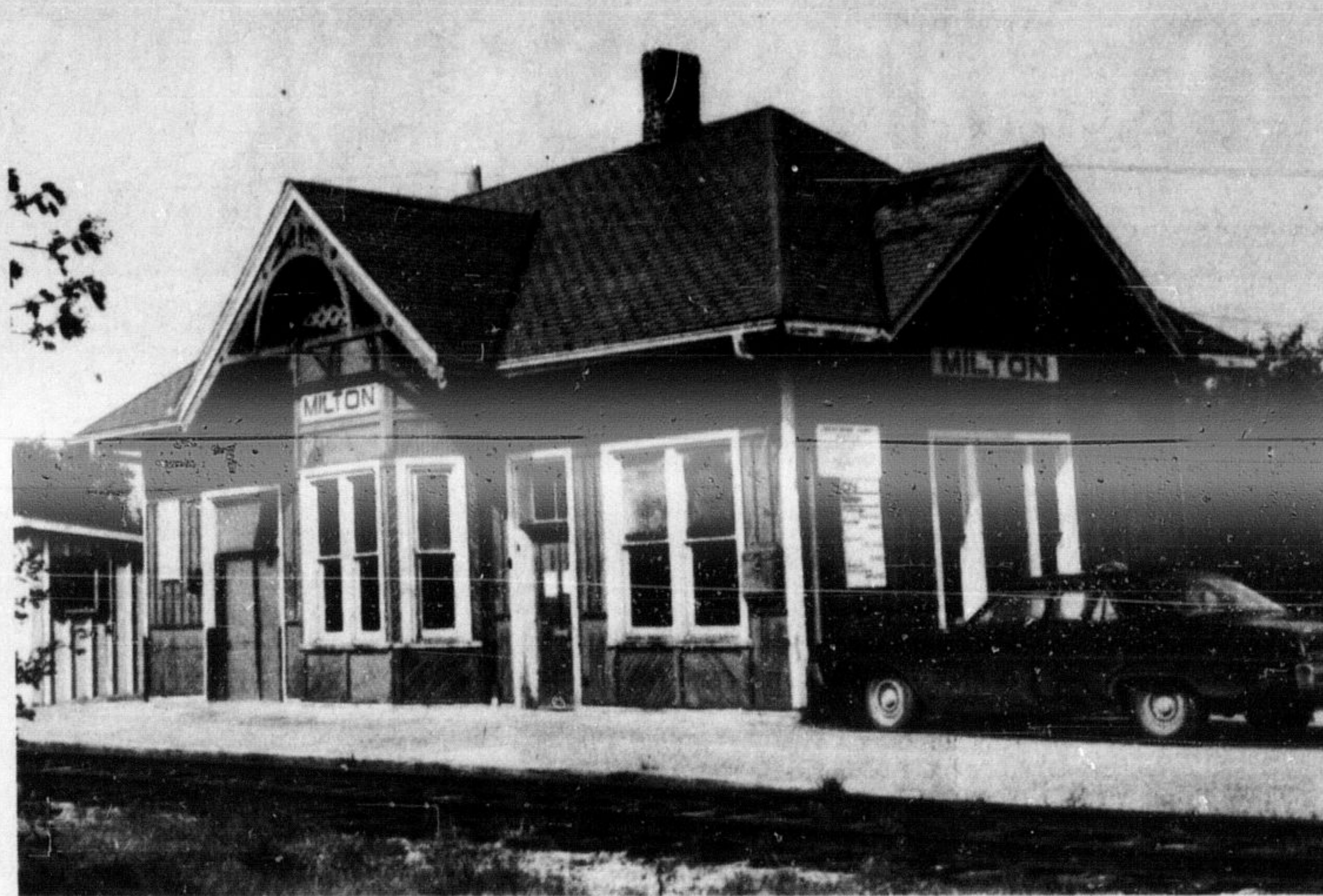
MILTON'S C.N.R. STATION on Bronte St. has served its last train passengers and freight. A final order closing the station, removing the agent and authorizing the removal of the building were passed recently by the Canadian
