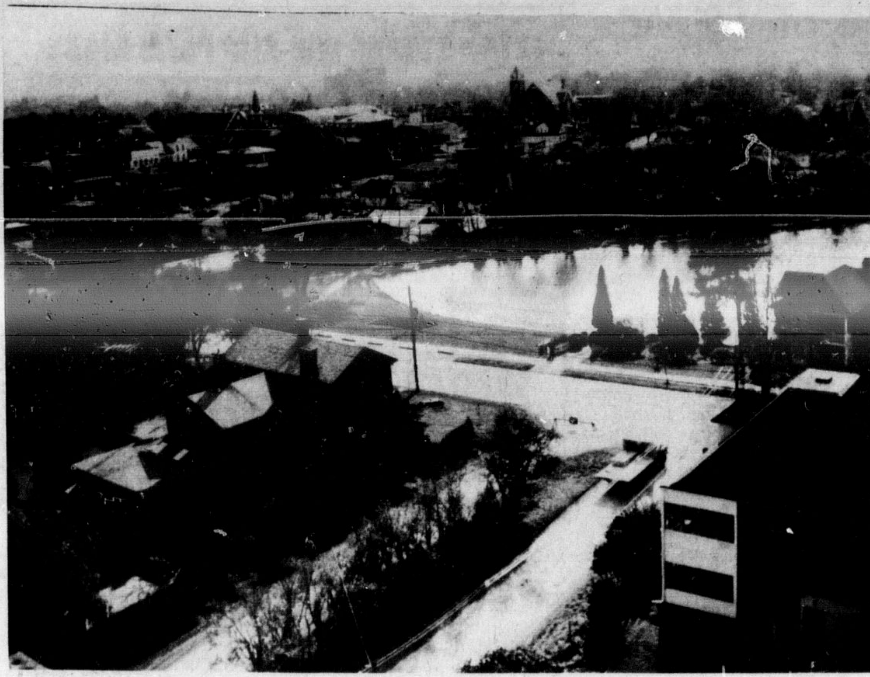
THE POND FROM ON HIGH... Construction of the 11-storey Noble Towers apartment building on Millside Dr. near Martin St. was too good an opportunity for photographer Jim Jennings to pass up. He climbed to the roof one day recently to get a bird's eye view of
