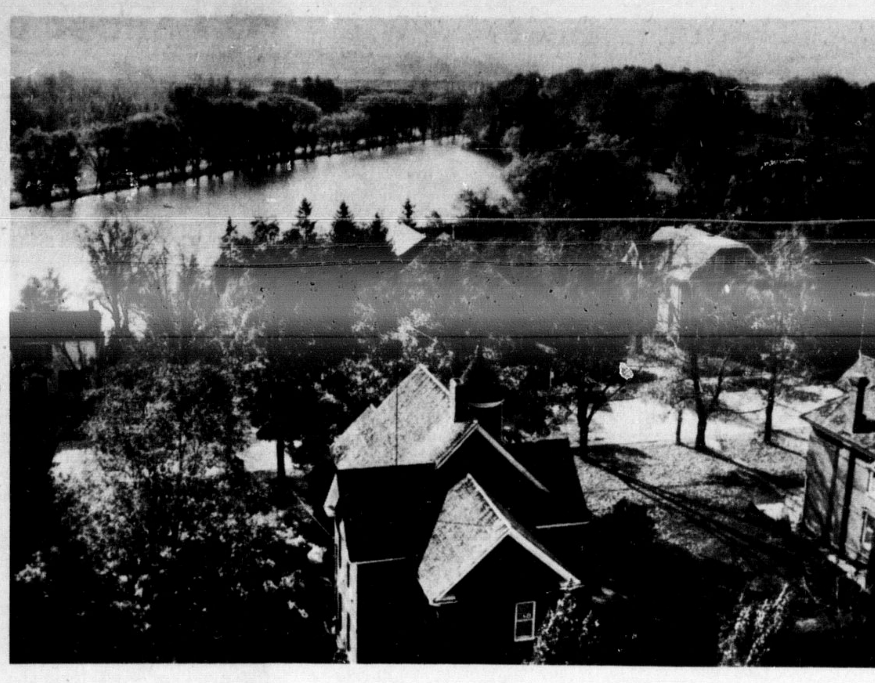
central part of Milton and on this page are some of his photos from that lofty perch, as future tenants will see it. Above, the mill pond glistens in the afternoon sun.
