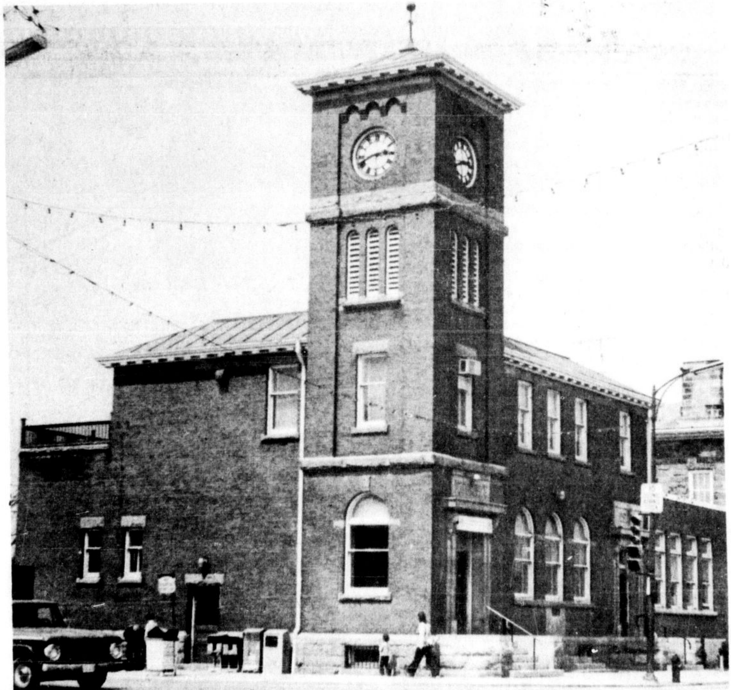
MILTON'S POST OFFICE, which has occupied a place of prominence on the corner of Main and Martin Sts. since 1916, may not be there much longer. Halton MP Rud Whiting announced this week a feasibility study is being undertaken right away, on
