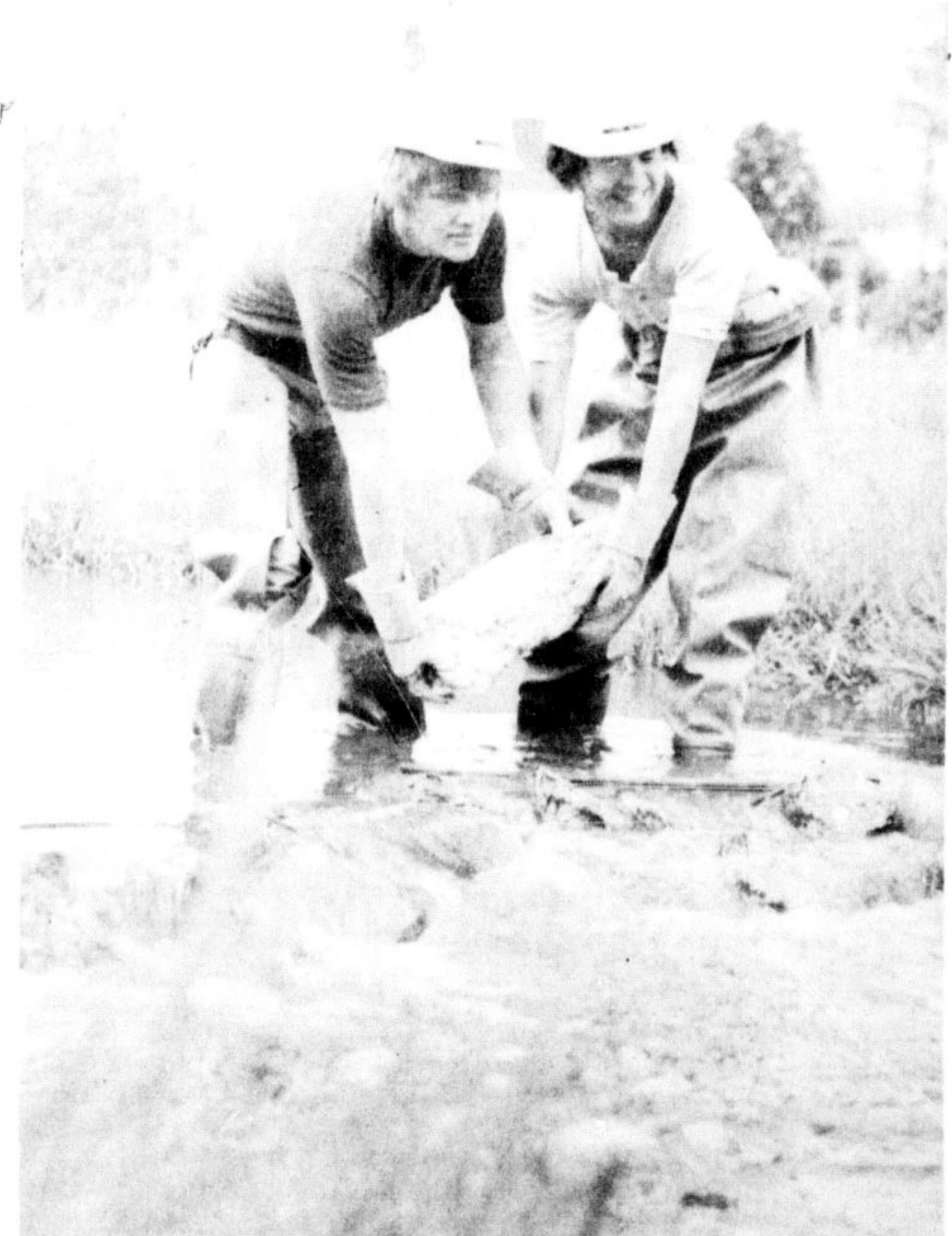
TOSSING ANOTHER STONE into Sixteen Mile Creek, Kevin Nye and Wayne Allison are not polluting the creek but rather helping it with its flow. Step-stone dams are being built by SWEEP workers to increase the oxygenation of the water in the creek. See Page 12.—(Staff Photo)
