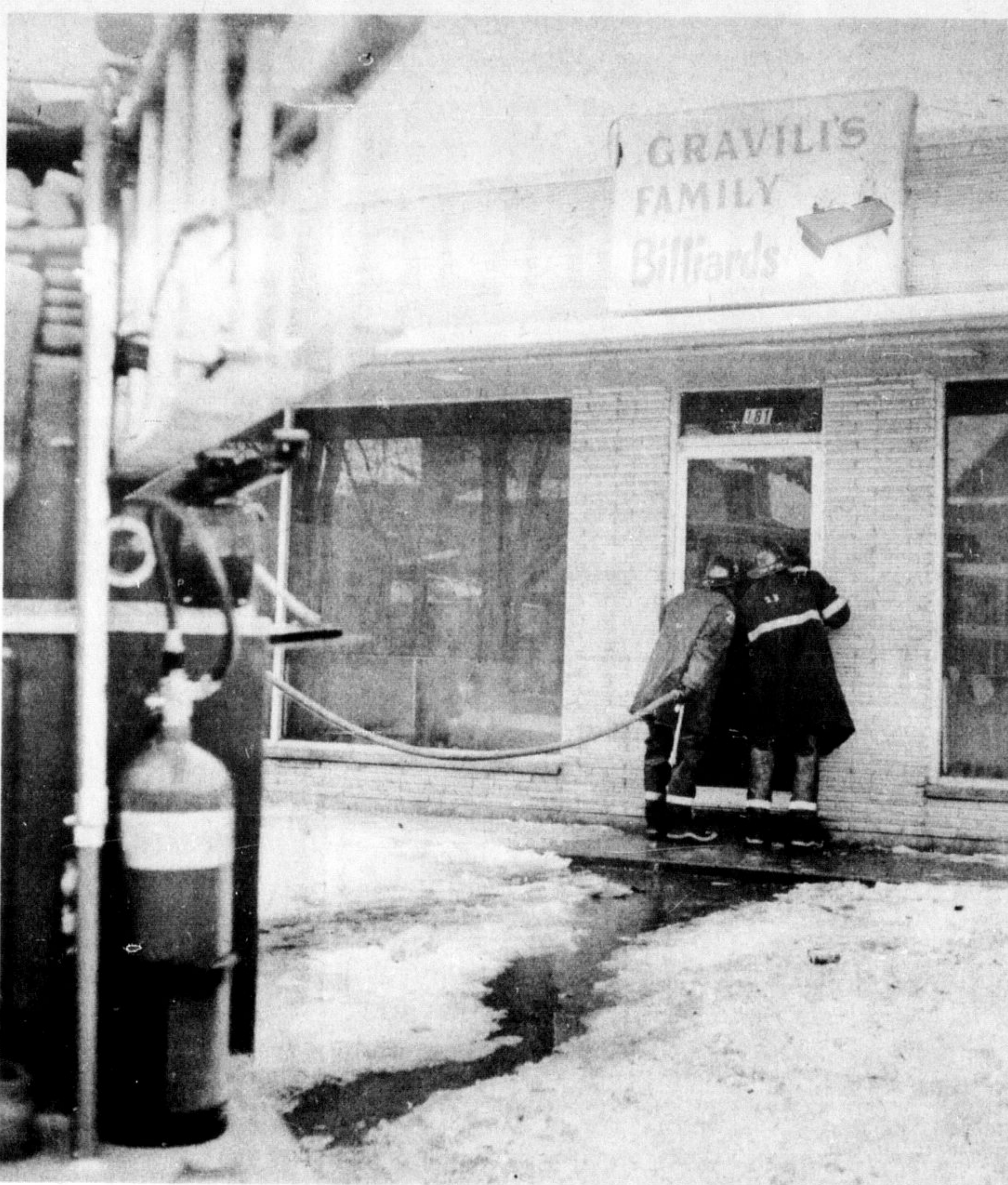
CHRISTMAS MORNING FIRE , believed to have started in a car racing machine, did an undetermined amount of damage in the Mill St. Gravilli's Family Billiard room. The fire started on the west wall of the building about the middle of the side and burst a hot water tank nearby. Milton Firefighters were called when Sgt. William Patterson noticed the smoke filled building, while he was patrolling the area. Damage to the pool tables and the interior of the building had not been estimated at press time.—(Staff Photo)
