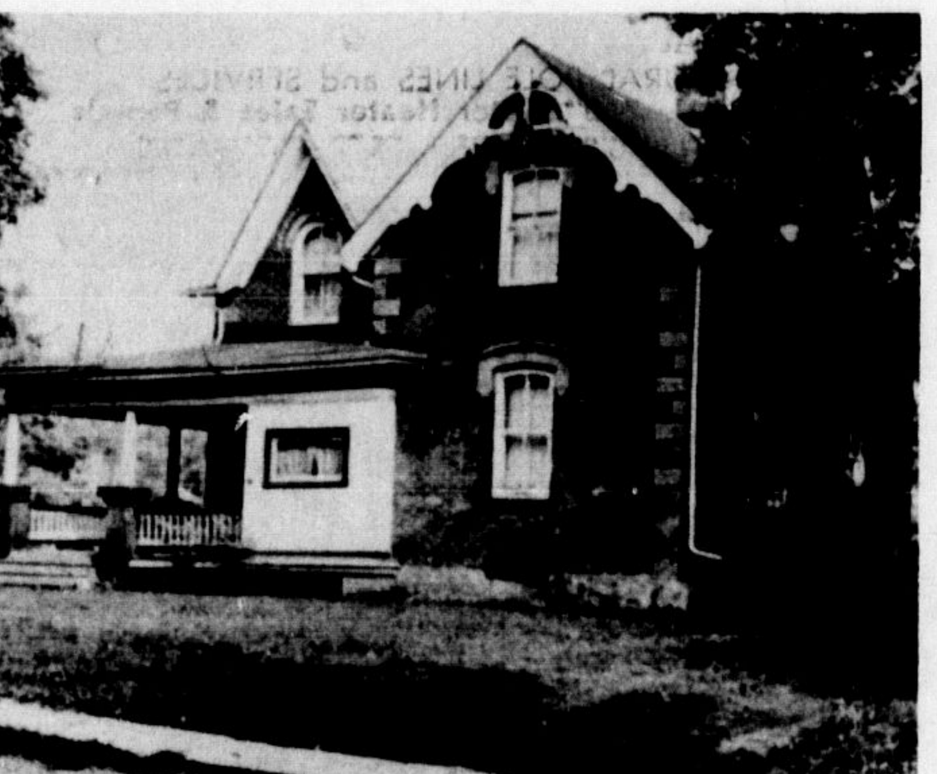
Investment special—ideal for conversion into a duplex—centrally located in Milton on a 66' x 132' lot. This home has 10 rooms including 5 bedrooms. Total floor area 2253 square feet—spacious rooms on the main floor—estate sale Listed Price $24,000.00 Mortgage—Funds can be arranged.
