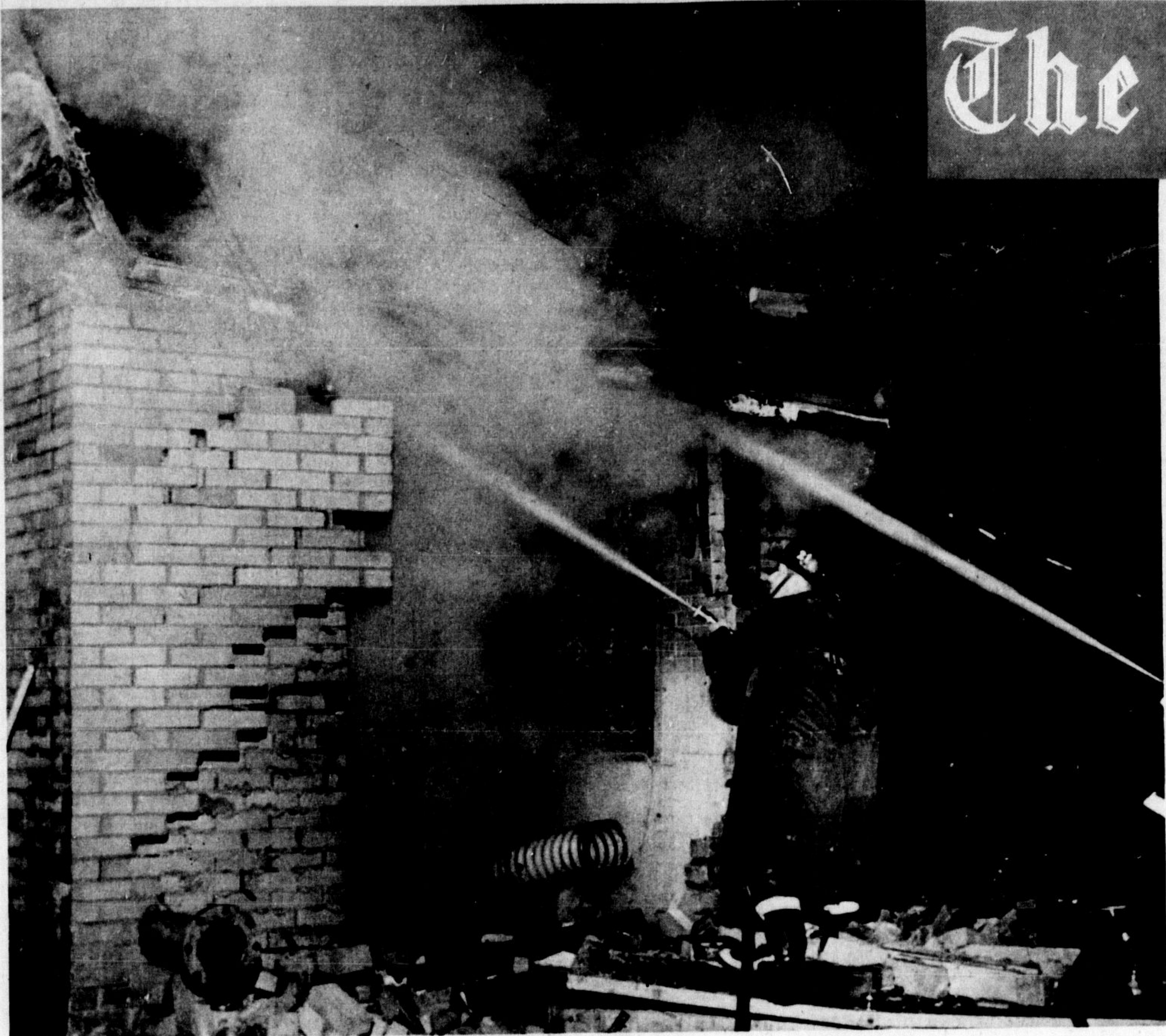
ONE PERSON WAS INJURED and the solid masonry walls were destroyed when an explosion at the Robert St. pumping station rocked the area early Sunday morning. The force of the blast blew out the masonry walls and raised the roof of the small building. Firefighters are seen here controlling the fire that followed the explosion.—(Staff Photo)
