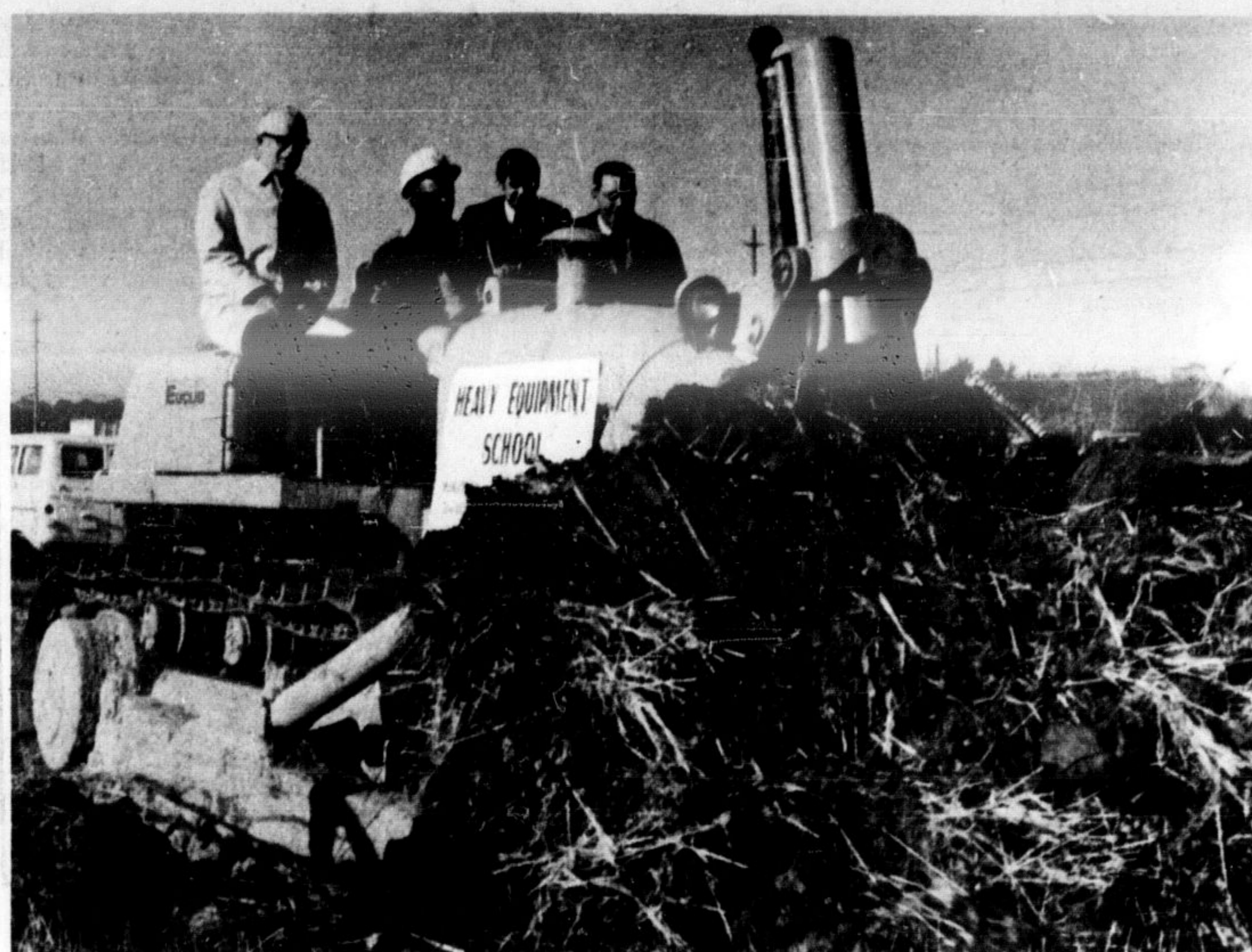
THIS IS SOD TURNING in a big way. Archie Turner, Chairman of the Board of Governors for Sheridan College, George MacDonald an instructor at the Heavy Equipment School, Bryan Frank, president of the Student Senate and J. M. Porter, president of the school go along for the ride on the sod-shoving dozer at the ceremony on Trafalgar Road Monday. (Staff Photo)
