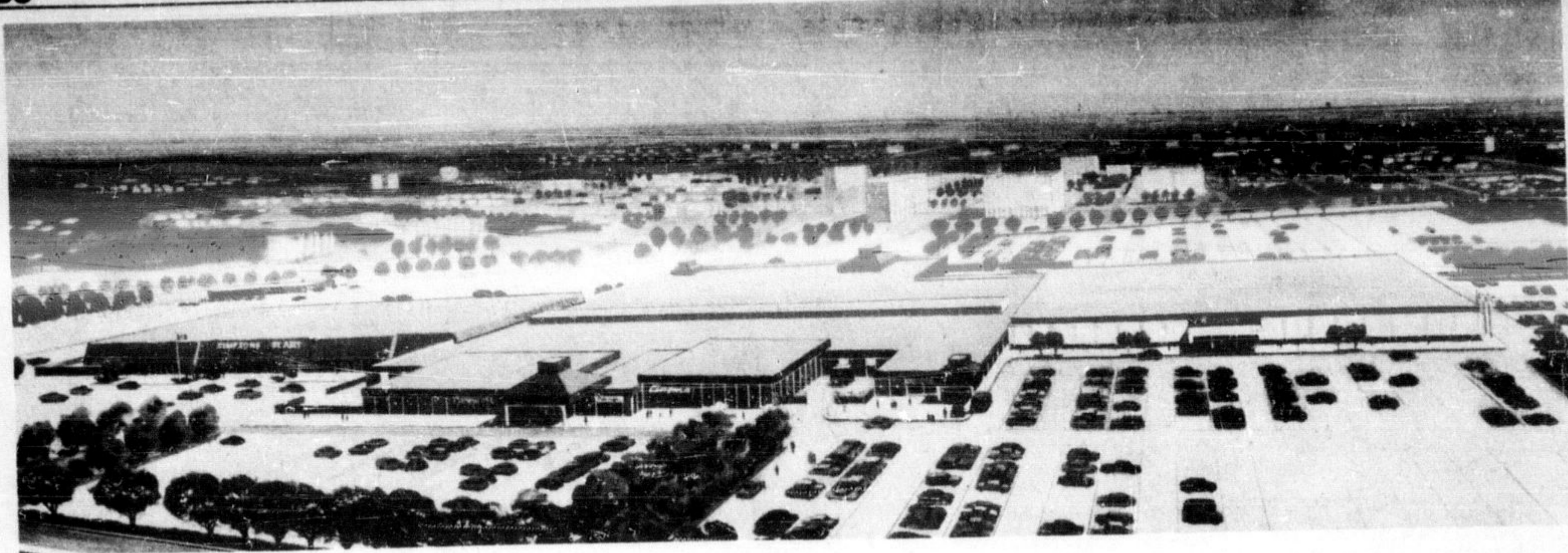
A $12 MILLION SHOPPING MALL is under construction on Burlington's Guelph Line just south of the Queen Elizabeth Highway, and should be open by October. Called "Burlington Mall" it will be an enclosed all-weather shopping centre with probably over 1,000 employees and parking for 3,400 cars.
