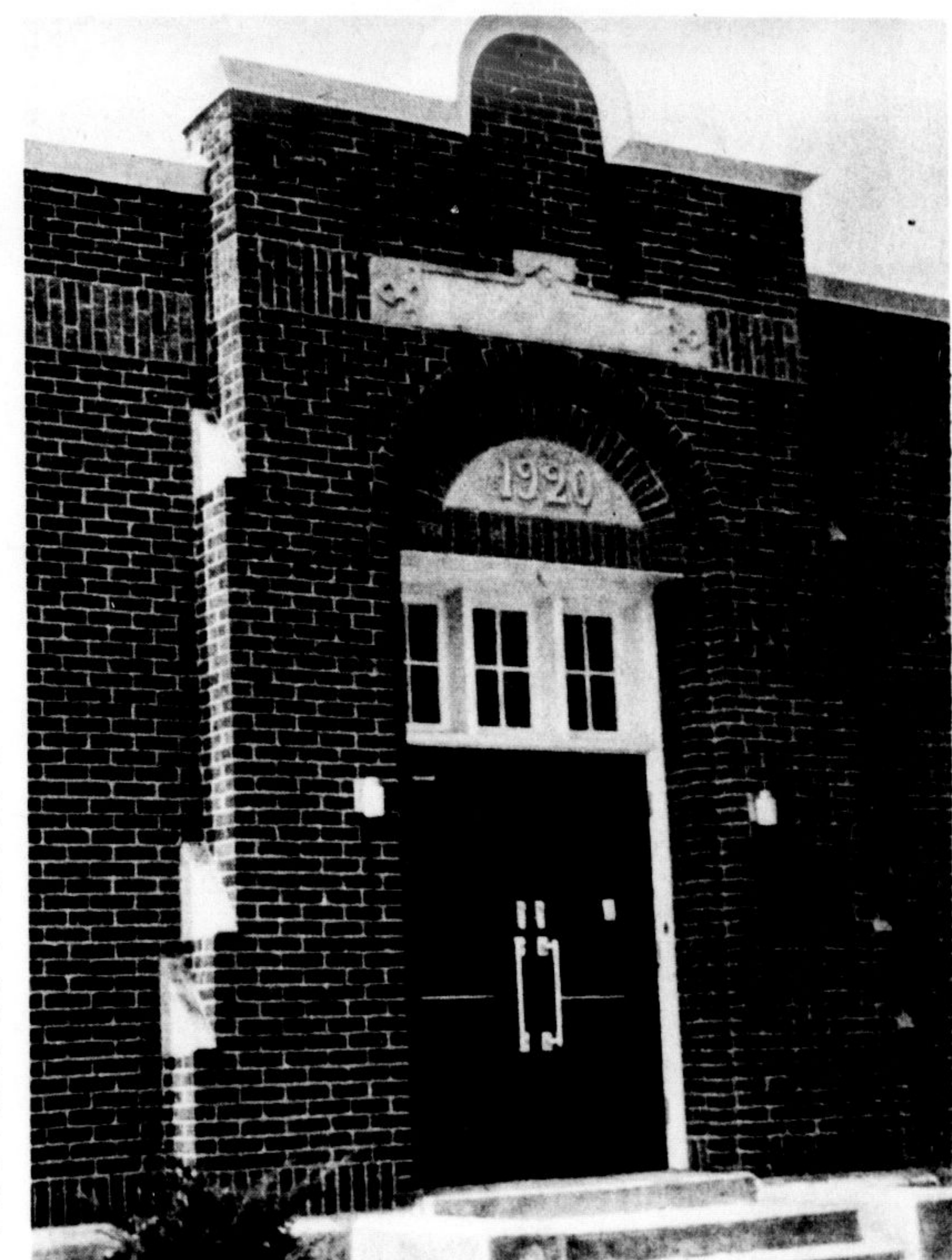
MARTIN ST. SENIOR PUBLIC SCHOOL in Milton is ready for the back-to-school influx of students, which takes place next Tuesday morning. All Grade 7 and 8 students in Milton will attend classes in this building, which was the former high school. School officials expect 264 students next week in this school. (Staff Photo)
