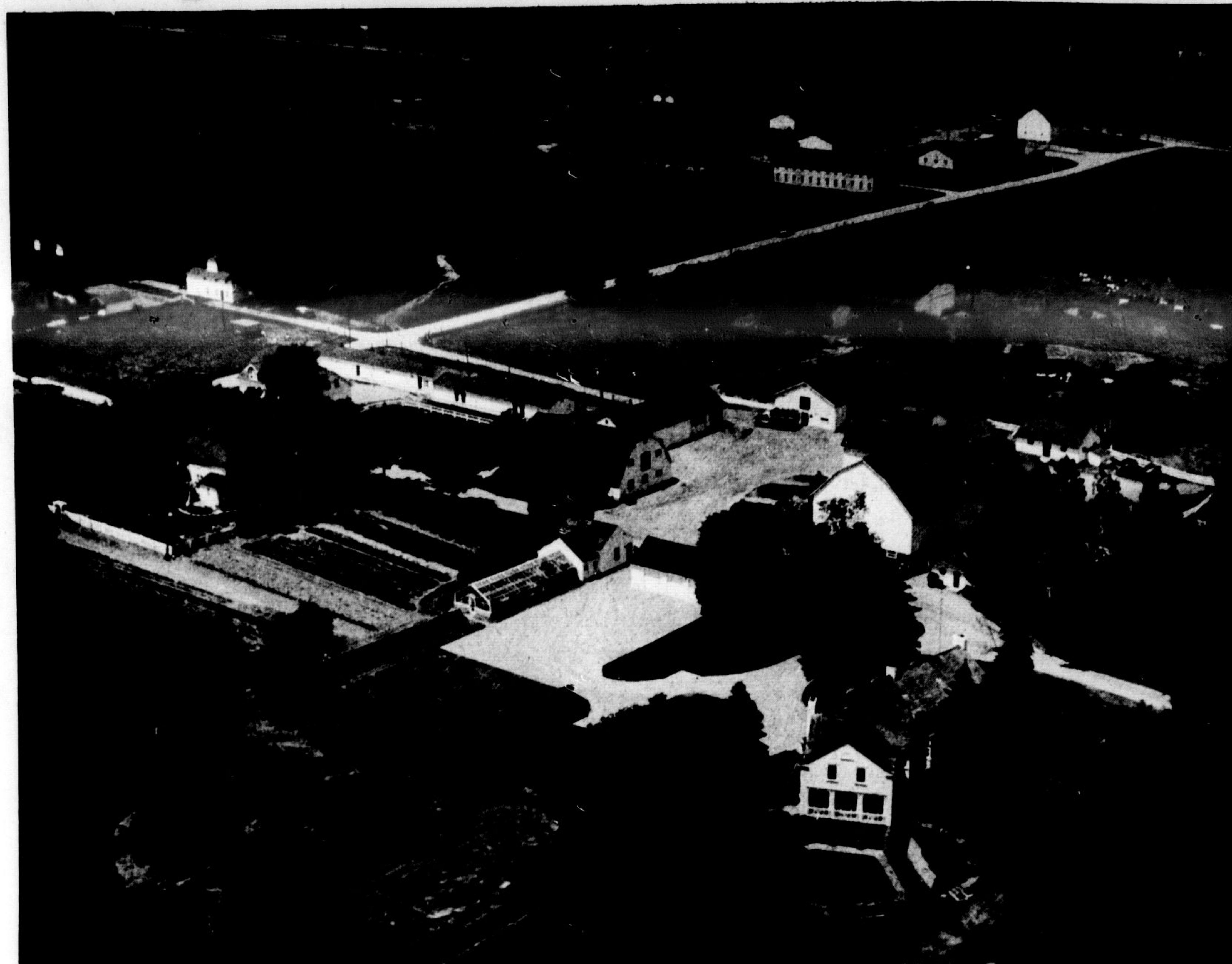
THE PRESENT RESEARCH FARM operated by Master Feeds near Thornhill is a sprawling complex of buildings — some original farm buildings that stood when the farm was purchased in 1937 and some new units added in more recent years. The firm is "phasing out" the Thornhill farm and transferring its research operations to the Hornby district farm, beginning next spring. (Photo by W. J. Watson)
