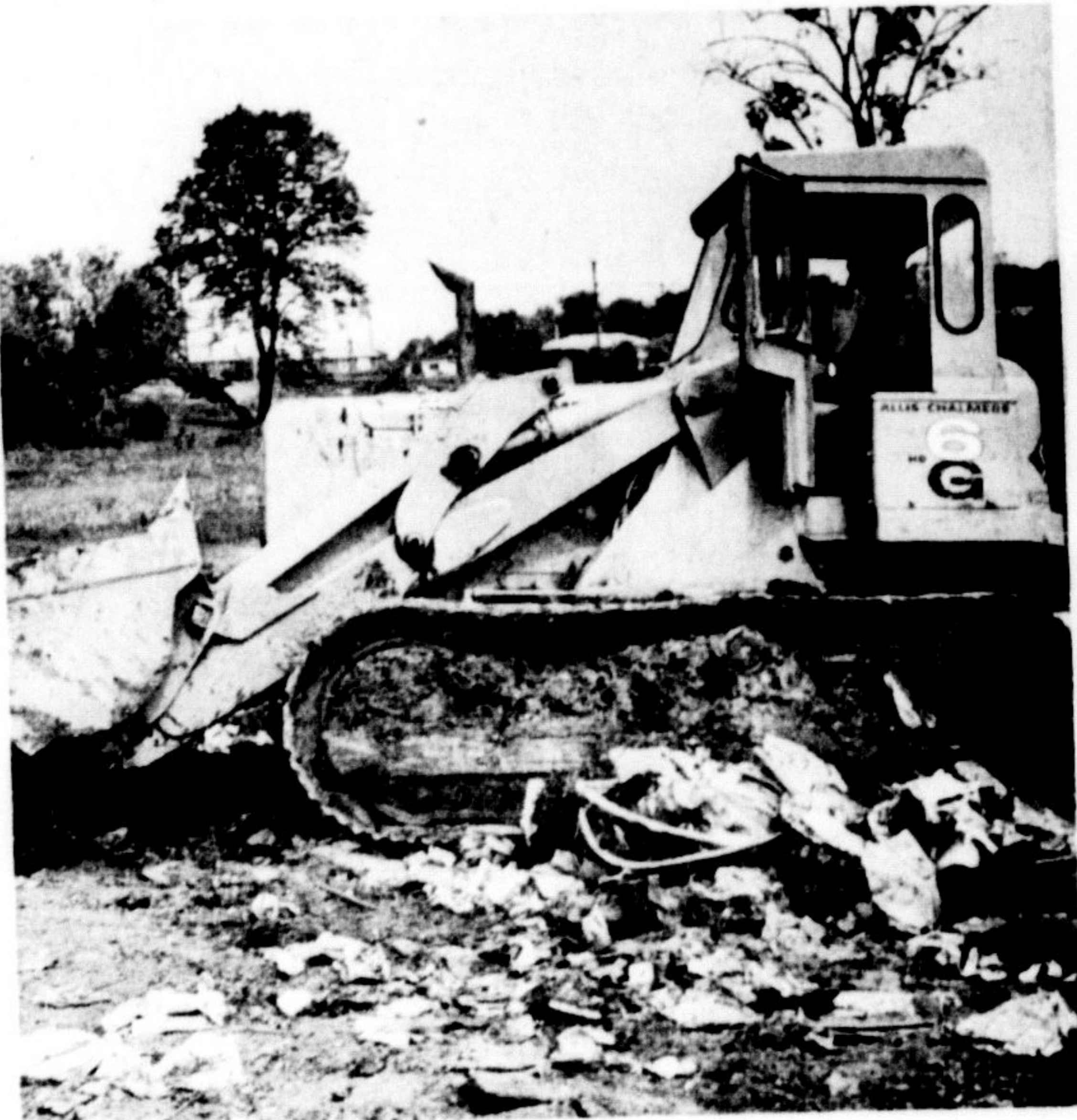
OPERATOR DICK VEENSTRA COMPRESSES REFUSE BEFORE BURIAL
