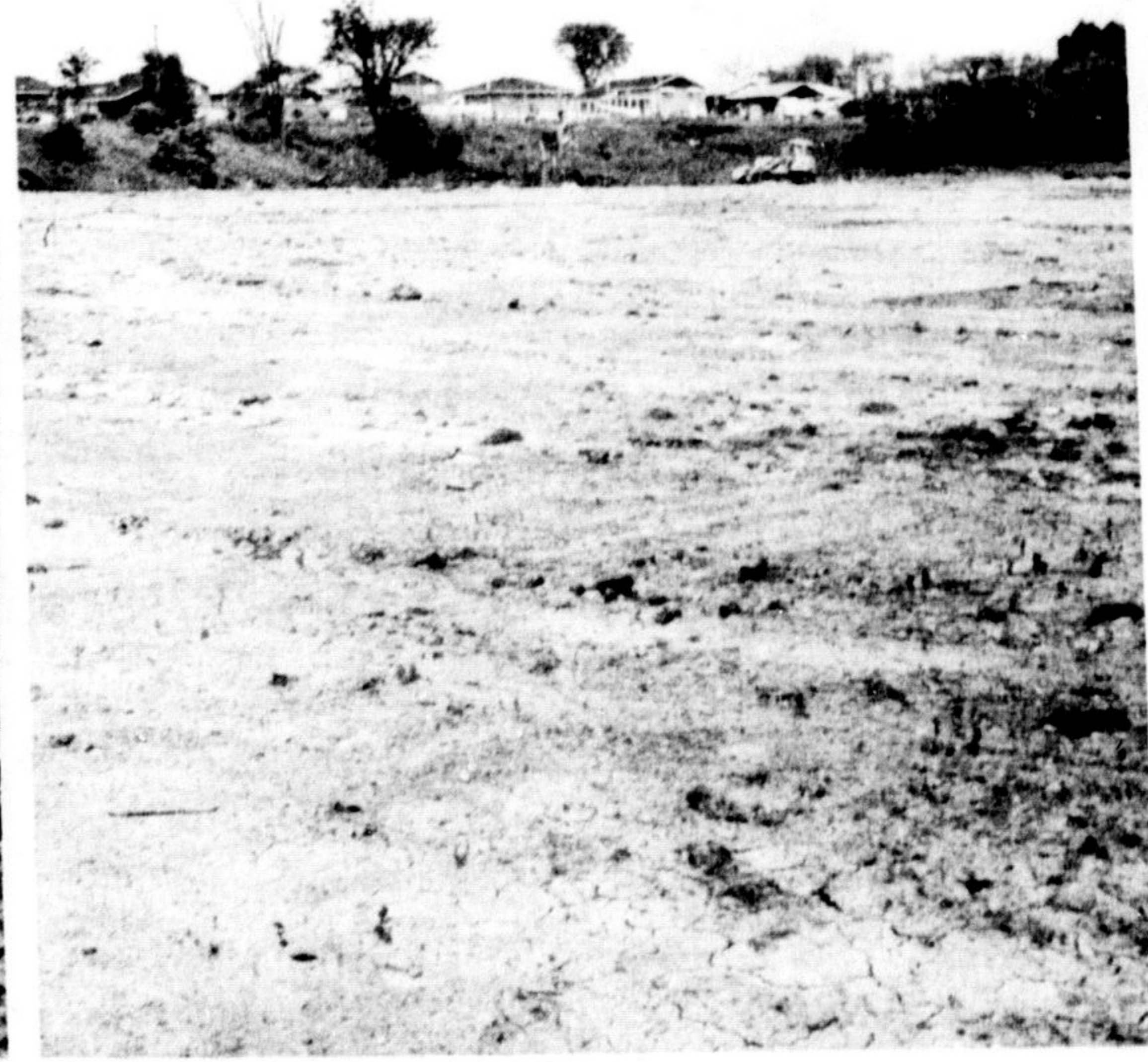
SURFACE IS CLEAR OF DEBRIS ON COMPLETION
