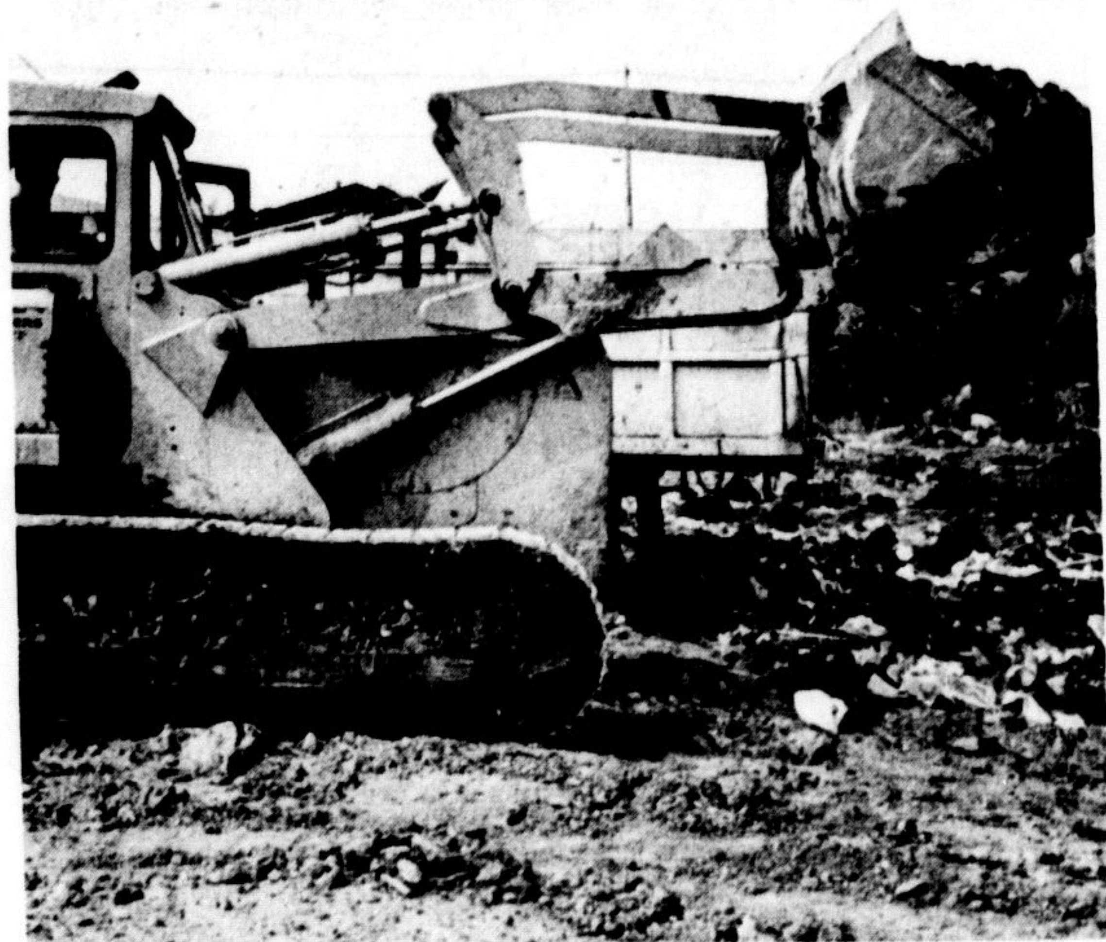
FILL IS SPREAD OVER REFUSE
