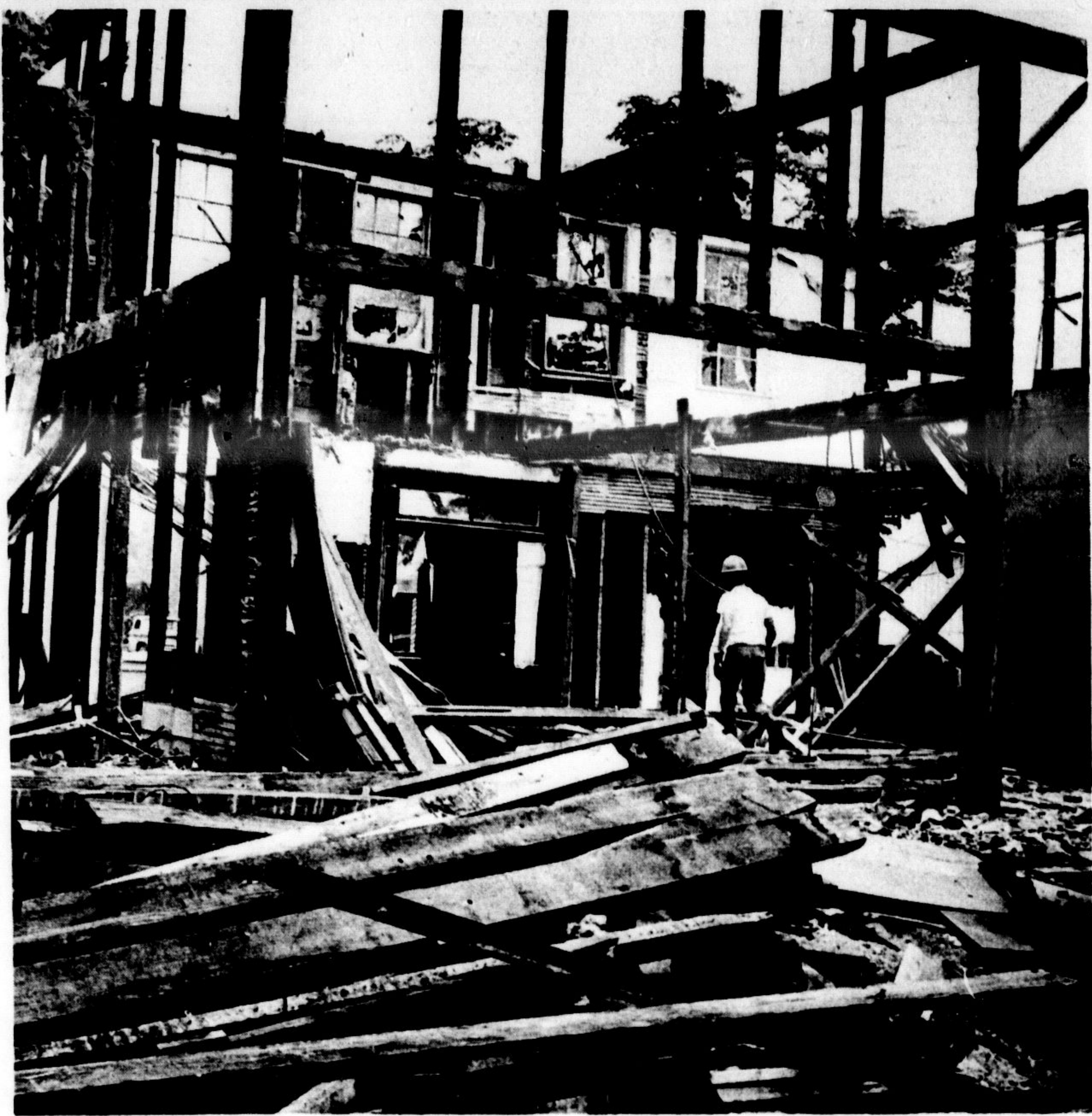
PROBABLY OVER A CENTURY OLD , the old house at the Martin-Mill Sts. intersection that until now has blocked the view of Milton's beautified mill pond centennial project, is no more. Harry Herensberger and a crew of men have wrecked it and removed it from the site, to allow landscaping and gardens to be added along the Martin St. end of the pond. The old beams were notched together and some old square-headed nails were found in portions of the house. This is how the house looked on Friday just before the workmen finished stripping off the salvage and pushed over the remaining framework. (Staff Photo)
