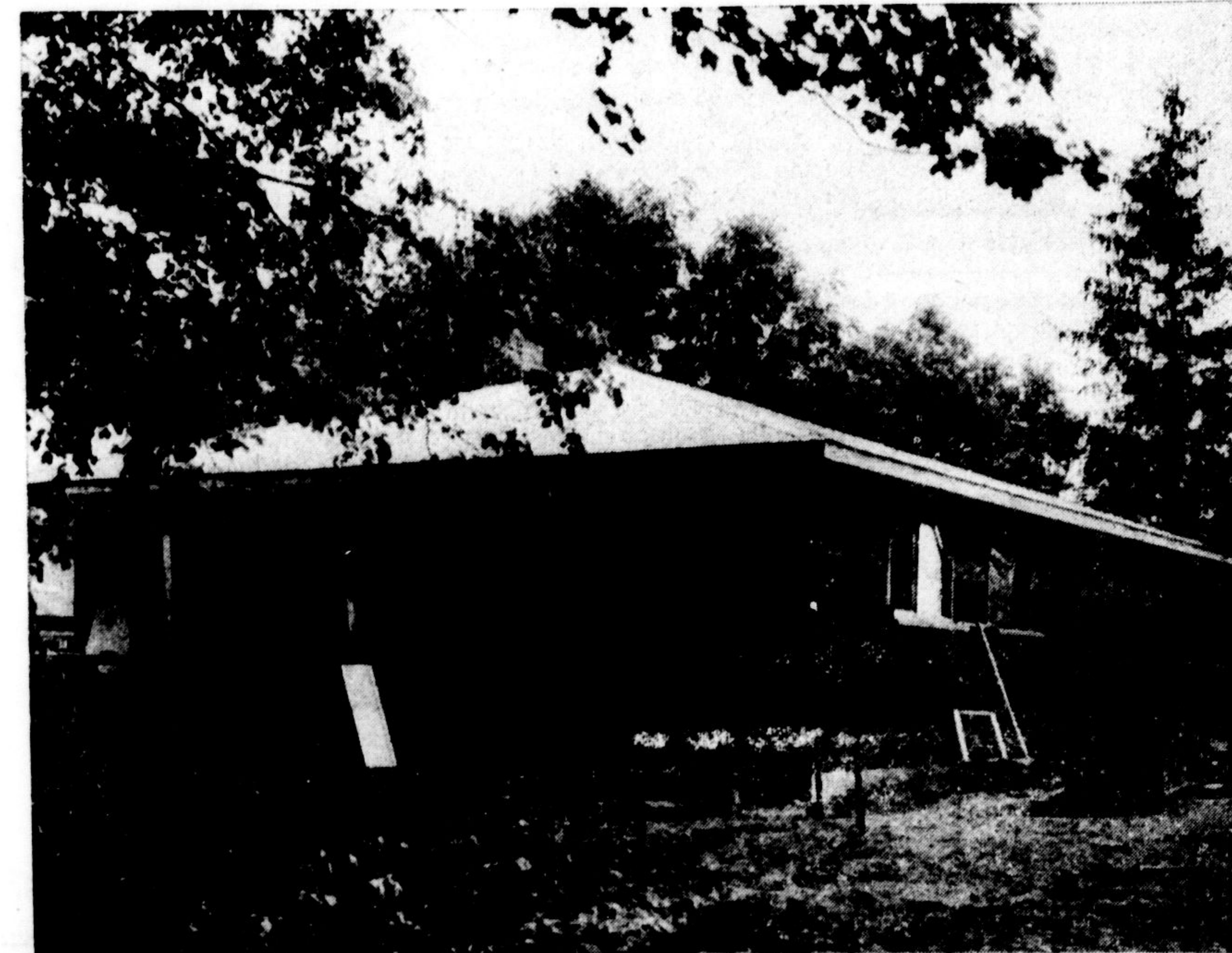
HOUSE CONSTRUCTION IN MILTON has slowed off this year and local realtors report, in a special Champion feature this week, that the housing situation is reaching the critical stage. This house being erected on Sydney St. is one of just eight built in town this year. Realtors report a growing demand for accommodations in town, and there is very little to offer them.
